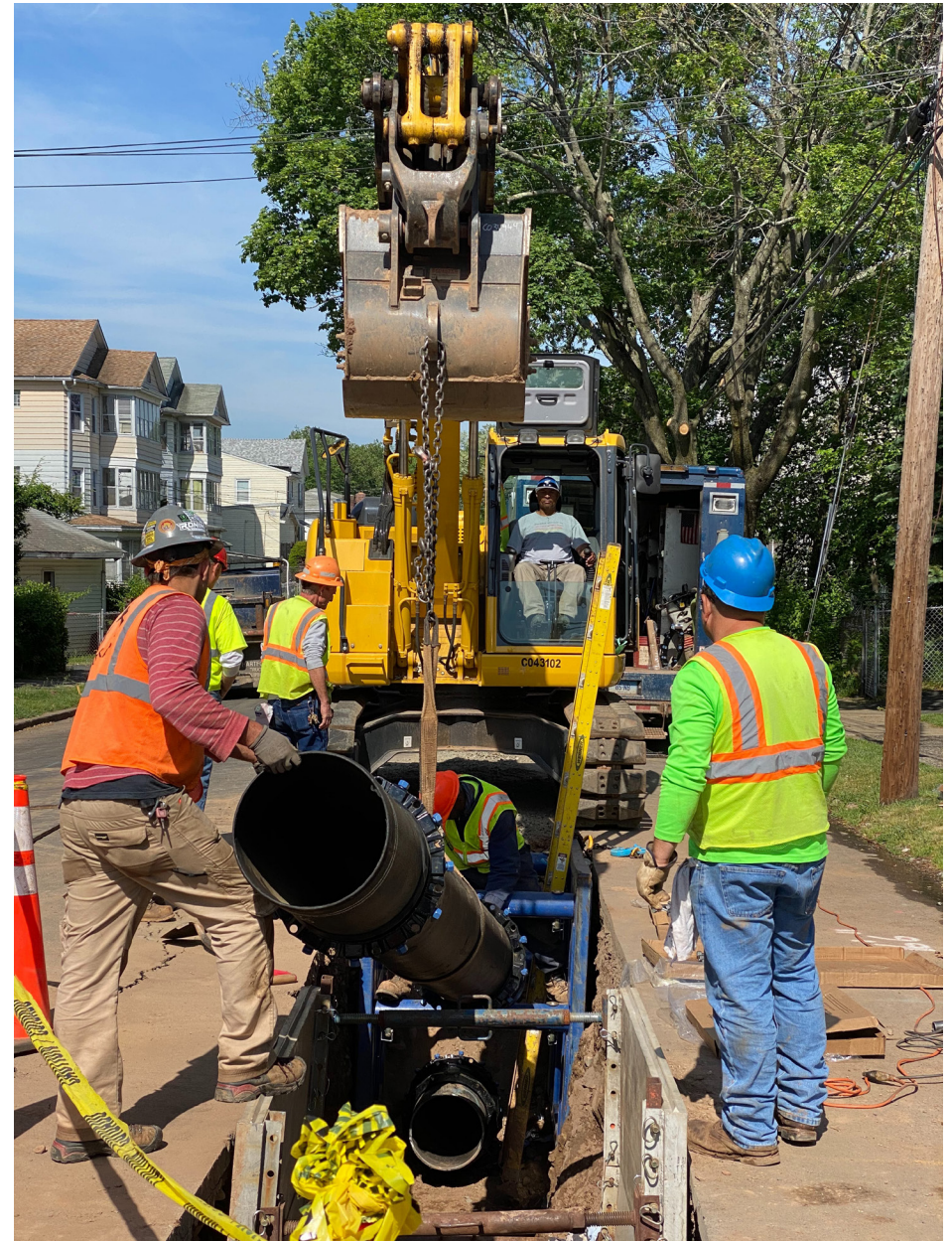
Water line replacement on Broad Street
