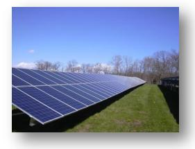
The array is located on 2-plus acres of land and is made of 16 rows which hold 2564 panels. These rows are arranged
