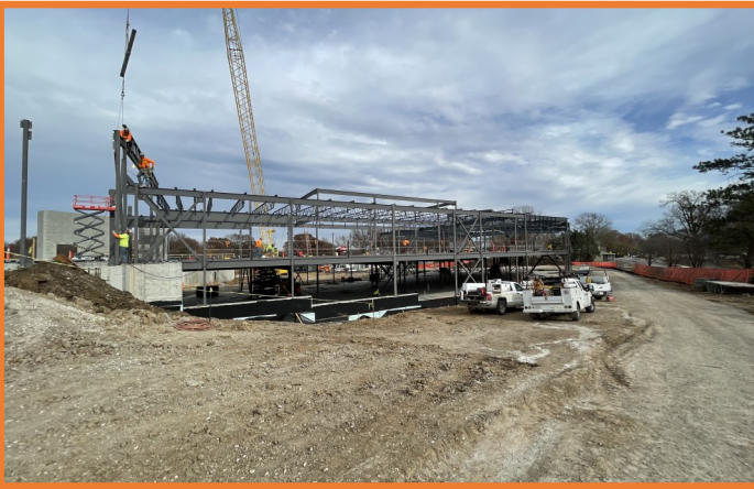
Area C Structural Steel Progress
