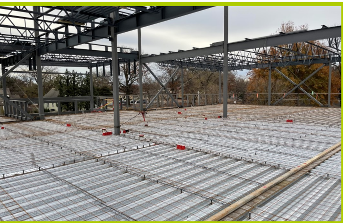
Area C Slab-on-Deck Prep
