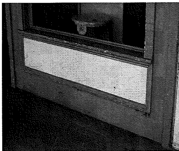
The building at 44 Main Street retains its original frame bulkheads. This historic storefront element should be maintained.
