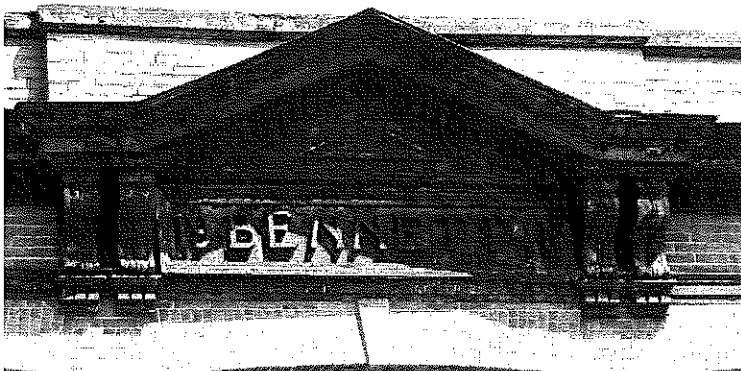
This metal cornice is not severely damaged, just in need of cleaning. Repair is recommended over replacement.
