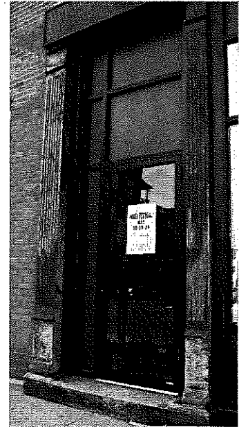
These original cast iron pilasters at the entrance on 191 Arch Street should be retained and maintained with gentle cleaning.
