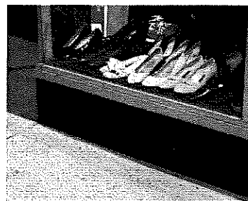
The photo below shows the same building's bulkheads with Carrara glass.
