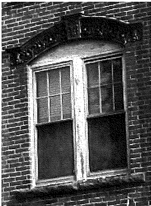
Non-abrasive methods will carefully remove flaking paint, then fresh paint can be applied. (116 Winter Street)
