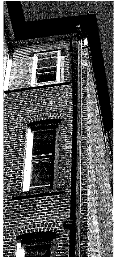
This downspout helps contain rain water and diverts it away from the building at 66 W. Main Street.
