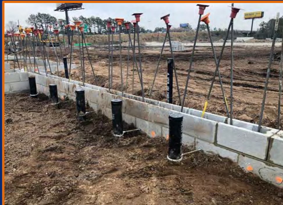
Underground Plumbing at Concessions
