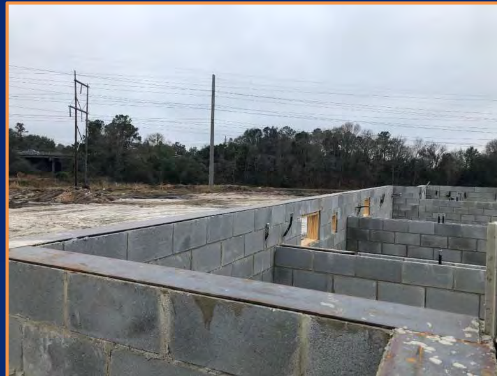
Embed Plates Installed at Field House
