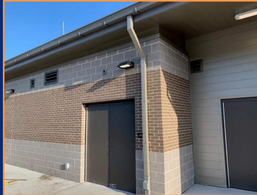
Downspouts Installed at Field House
