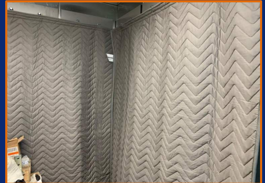
Quality Spotlight: Elevator Cab Installed and Protected
