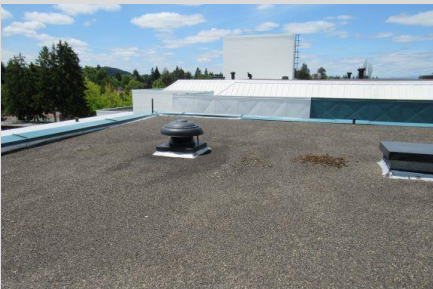
moss build up and drainage issues
