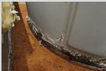
corroded water heater
