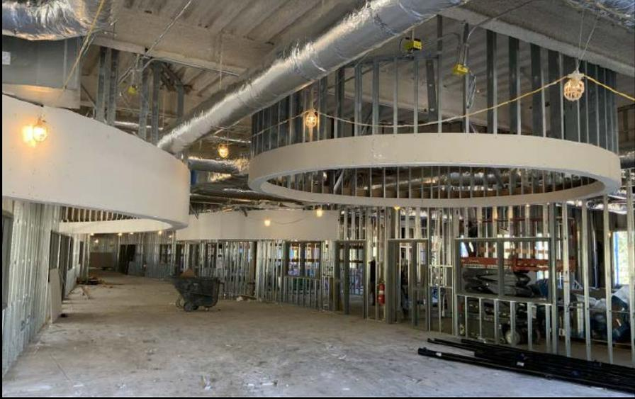
Installation of Main Duct Line, Metal Studs at CMU at Food Service Area, Spray Fire Proofing to Roof Structure, Interior Gyp. Bd. Fur Downs
