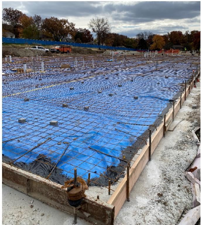
Area D Slab on Grade Prep
