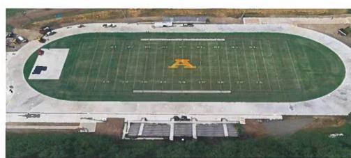
Concrete track surface and new artificial turf
