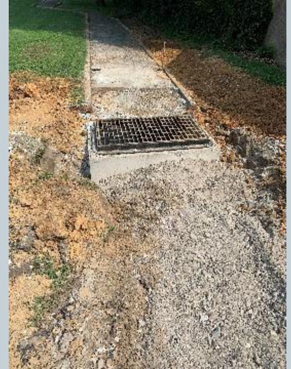
Oakmont Storm Drain
