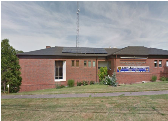
Solar panel installation at the Vernon Police Department Headquarters
