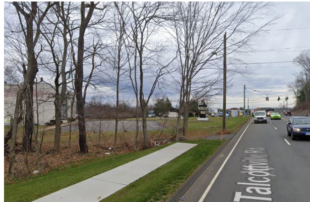
Sidewalks are required for all new development within commercial corridors, but was not required historically. This results in a disjointed sidewalk system
