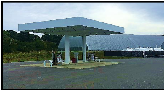
New Fuel Island with aboveground fuel tanks
