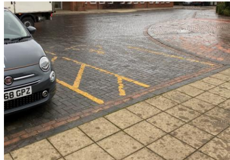
Repainting parking areas
