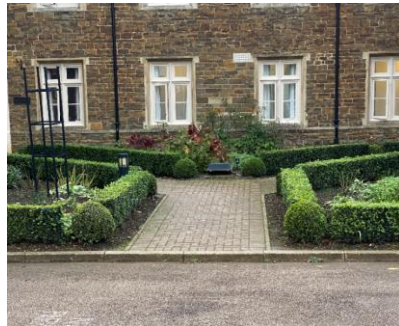
Drop Kerbs at GT / HT
