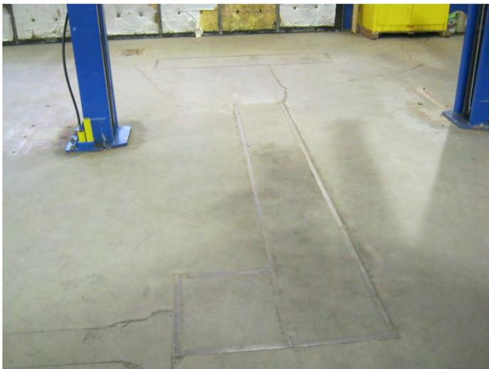
**In-ground hydraulic lift (one of four) in automotive garage.**
