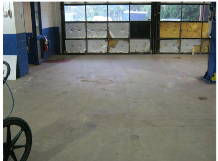
**Concrete patch at piston, with lines running north to the wall in southeast portion of automotive garage.**
