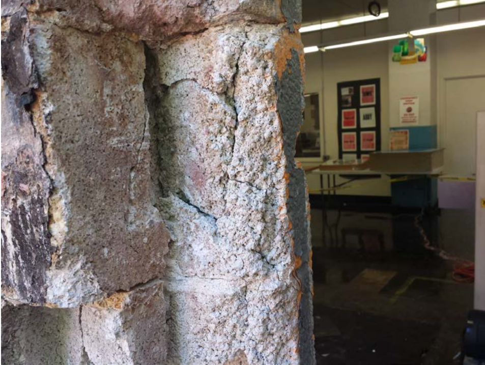
Photo C – deteriorated CMU
