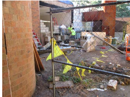
Photo G – wall being rebuilt.
