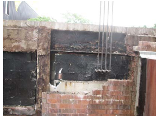
Photo S – area where CMU was removed
