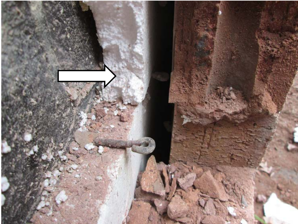
Photo L – South elevation; location one – east side of test cut; view showing the eyehook beyond without the pintle.
