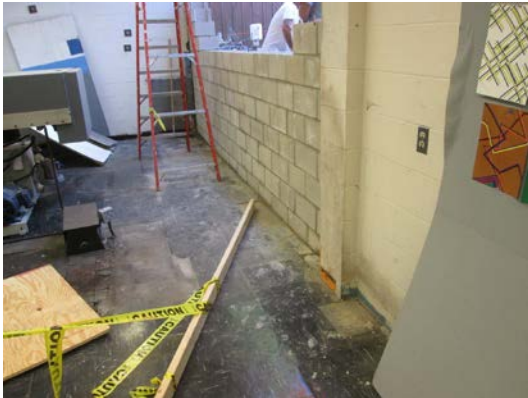
Photo F – wall being rebuilt.
