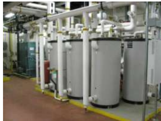
Water Heaters Fed from Boilers
