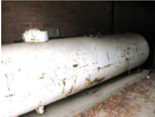
Generator Propane Tank
