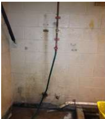
Hose Connection without Vacuum Breaker
