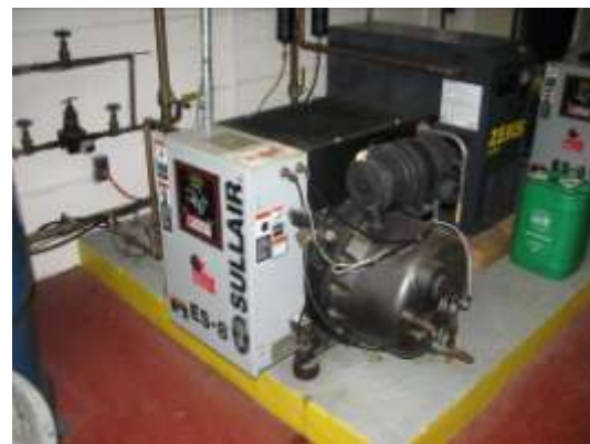
Duplex Air Compressors & Dryer
