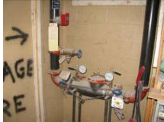
Sprinkler System DCVA & Flow Switch
