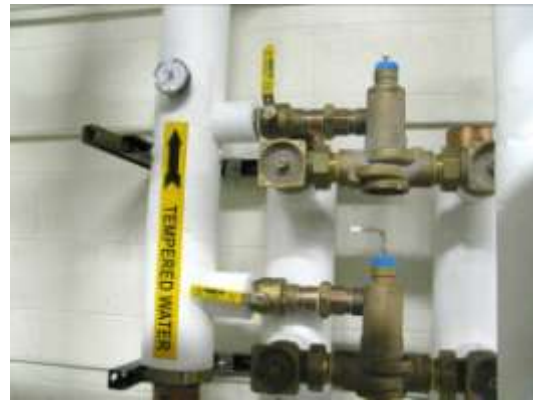
Domestic Hot Water Mixing Valves
