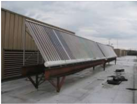
Abandoned Solar Collector
