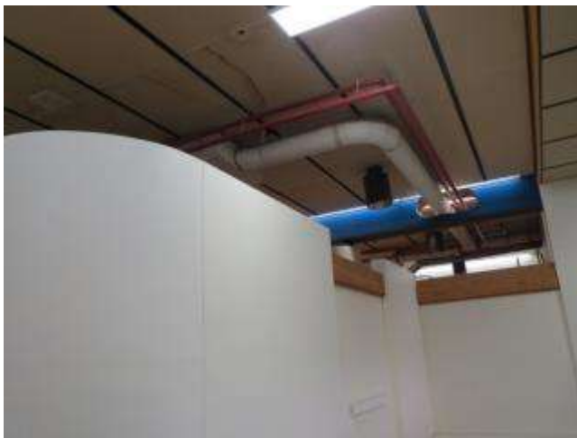
Culinary Arts General Area Conditions: There are unfinished ceilings, exposed piping, electric conduit and duct work render most areas almost impossible to maintain as a sanitary environment.
