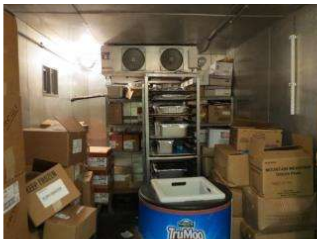
Walk-In Refrigerators and Freezers: Shelving is constructed of inappropriate materials; inadequate in quantity; overcrowded. Some, insulation at drain piping has deteriorated.
