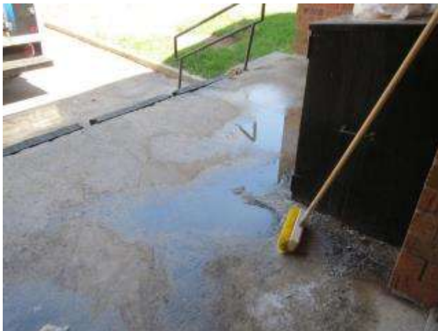
Receiving Exterior: Minimal water capture. Puddles throughout the area. Hazardous to foot traffic.
