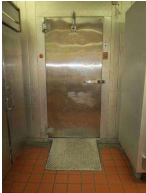
Bakery Walk-In Freezer: A portable exterior ramp is used to enter and exit, which makes it extremely difficult to transport mobile racks into the box; hazardous to foot traffic.
