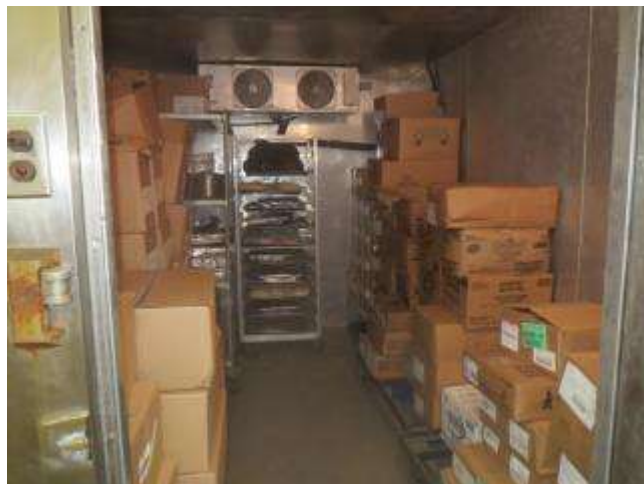
Walk-In Refrigerators and Freezers: Shelving is constructed of inappropriate materials; inadequate in quantity; overcrowded.
