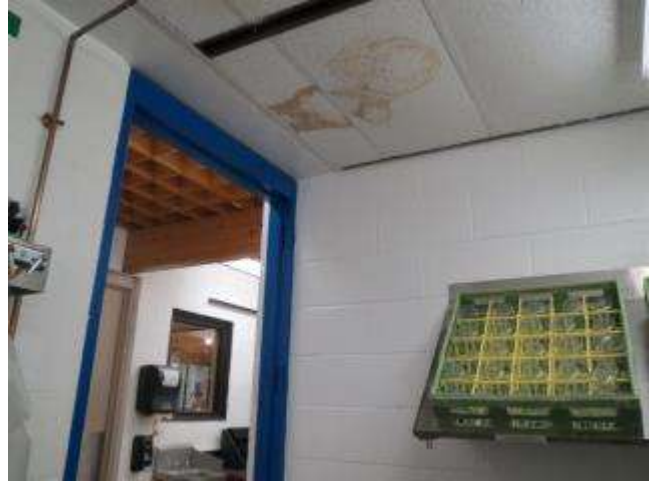
Culinary Arts Ware Washing Area: Perforated ceiling panels have degraded and are non-washable and therefore not code compliant.
