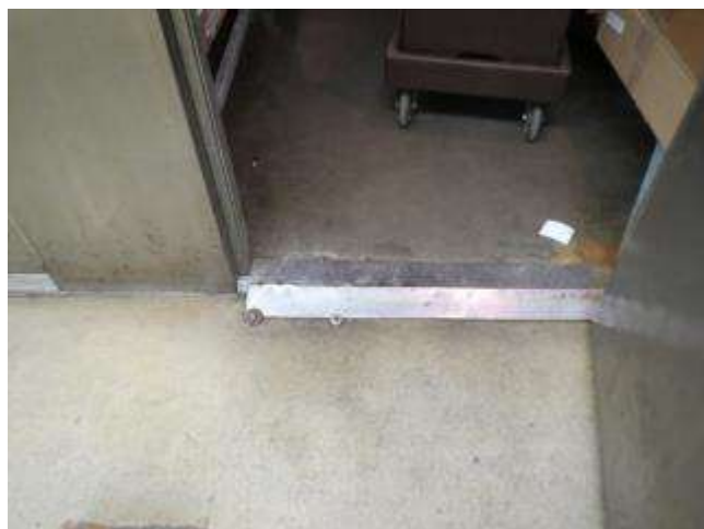
Walk-In Refrigerators and Freezers: Interior floor finishes and some door thresholds have degraded; unsanitary. Some areas are hazardous to foot traffic.
