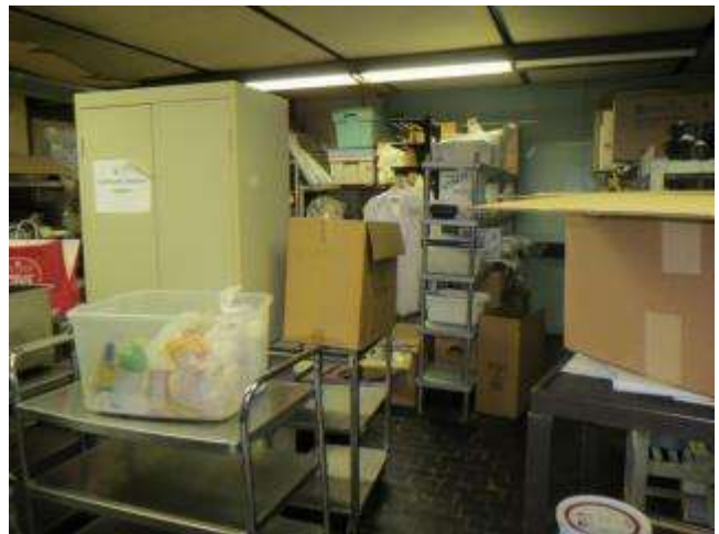
Dry Food & Paper Storage Room: Light fixtures lack protective covers and therefore not code compliant. Walls, floors and ceilings have degraded and are unsanitary.
