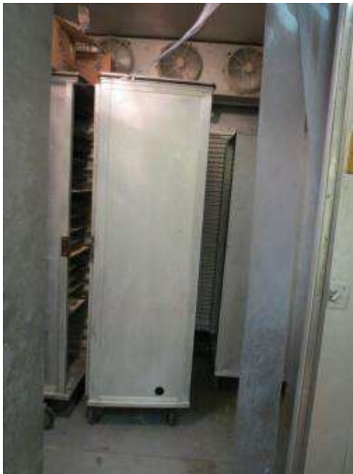
Bakery Walk-In Freezer: Interior floor finishes have degraded; unsanitary.
