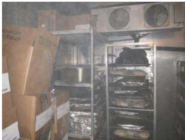
Walk-In Refrigerators and Freezers: Units are antiquated and undersized. Significantly overcrowded. Lighting is poor.
