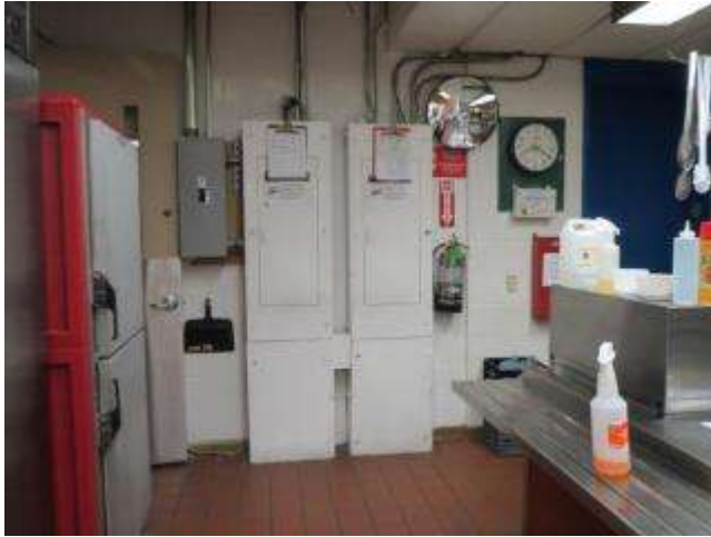
Culinary Arts General Area Conditions: Electrical panels, exposed piping and electric conduit render this area almost impossible to maintain as a sanitary environment.
