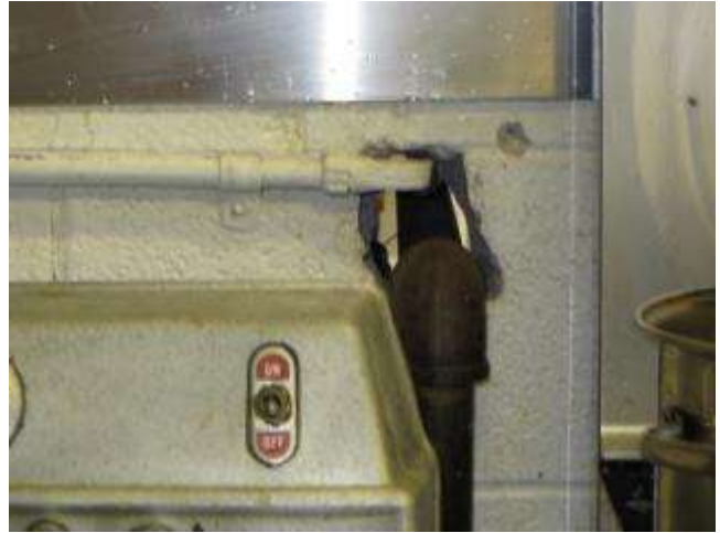
Culinary Arts General Area Conditions: Walls have degraded. There are open gaps in the wall at piping, which is unsanitary.
