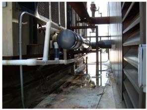
treatment is being provided for the cooling tower. The absorption chiller is a very uneconomical operating chiller which requires the steam boilers to run throughout the summer months to create the cooling energy required within the chiller. Consideration should be given to a complete upgrade of the chiller, however, the condenser water and chilled water piping and pumps are capable of being reused. It does appear that the cooling tower is in need of replacement.
