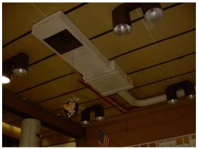
supply diffuser for providing ventilation and temperature air to each occupied area. All ceiling diffuses were noted to have surface soiling with overall condition consistent with their age of approximately 35 years.
