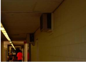
condensate and heat into an adjacent circulating corridor. This resulting condition is causing the communicating corridor to overheat and impose an additional air-conditioning load into this corridor. The entire condition should be upgraded.
