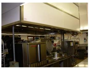
The exhaust hood is of the canopy style stainless steel design which is ducted directly through a dedicated exhaust system to roof mounted exhaust fans. The overall condition of the hood was noted to be good and clean and was provided with cleanable cartridge filters, and vaportight incandescent lighting.
