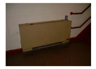
Communicating corridors throughout the entire building were provided with a limited amount of ventilation of which does not appear adequate to meet the current building code requirements. No exhaust systems were provided however should be considered to improve overall air quality.
