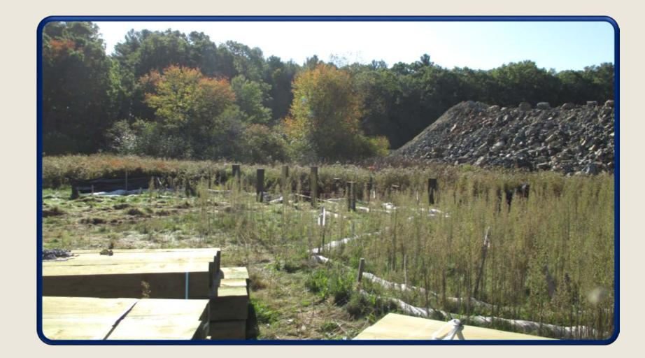
October 15th Timber Bridge C Installation of support piles.
