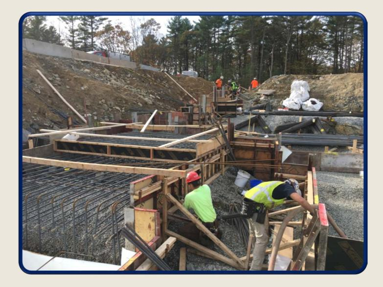
November 3rd View of Area C – Lower Level workers install rebar in the elevator and orchestra pit.
