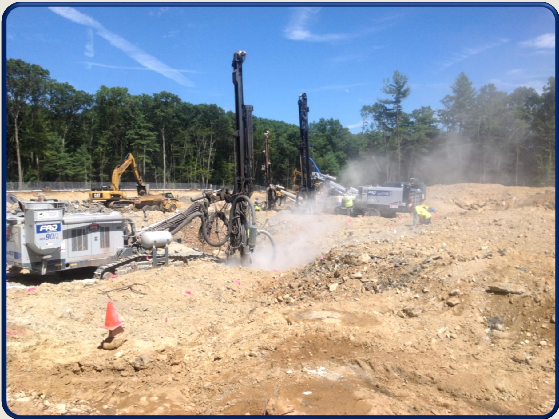
August 23 Northeast view of Drilling Operation
