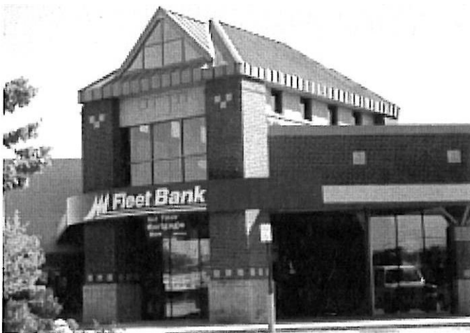
Main entrances on large-scale buildings shall be designed as prominent focal points to orient customers.
