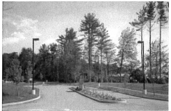
This curbed, landscaped island divides entering and exiting traffic. The identification sign is located away from the intersection to avoid interfering with the motorists' line of sight.
