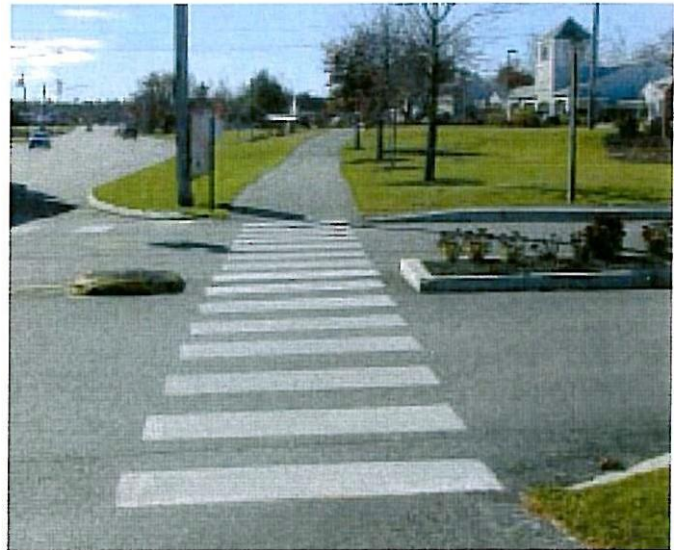
An island provides a refuge zone for pedestrians crossing this wide driveway. Permanent crosswalks would have minimized annual maintenance costs.
