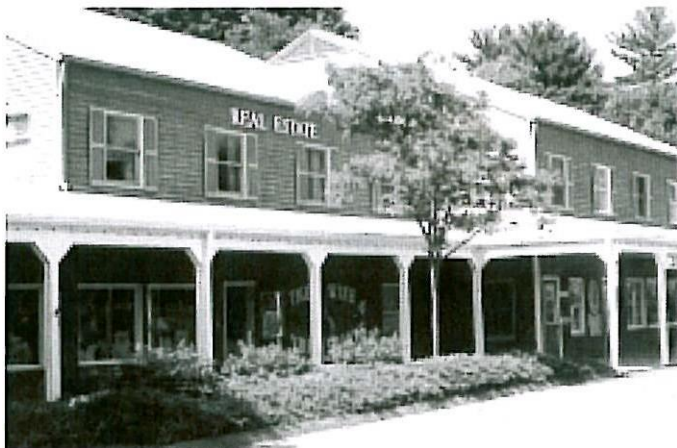
Covered walkways add a shadow line which can reduce the scale of a long building and unify the facade.
