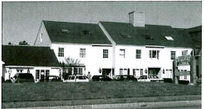
A low earth berm effectively screens a parking lot of Ornamental trees or plantings added to the berm would provide a greater degree of attractiveness, as well as separation from the roadway.
