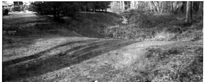
A stormwater treatment pond that is contoured to blend into the surrounding landscape.
