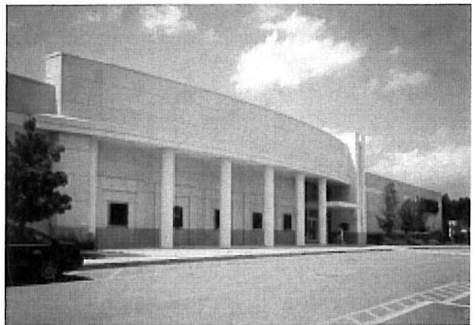
The mass of this large building has been reduced by a columns and subtle changes in geometry.
