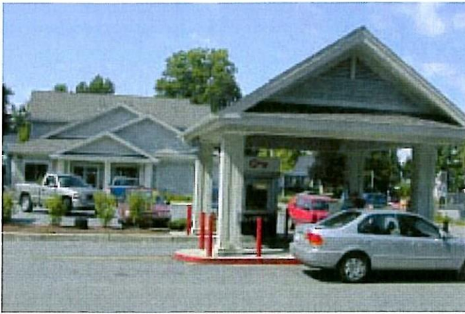
A free standing ATM and remote teller located in the rear of the building designed to complement the main bank building in color scale, and detailing.
