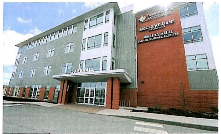
Examples of multi-story office, research and hi-tech buildings that have employed metal panels and brushed aluminum, coupled with brick and other traditional northern New England building materials.
