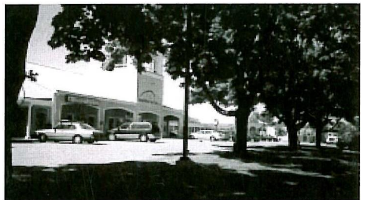
These mature maples were carefully saved during the development of this shopping area. The trees add character, visual interest, and shade.
