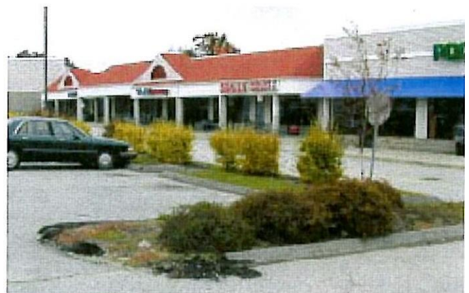
While asphalt curbing is inexpensive to install, it is very prone to snowplow damage.
