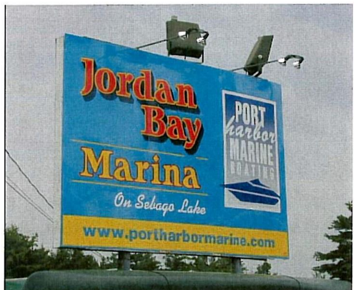
These top-mounted light fixtures are not well shielded nor integrated into the sign.
