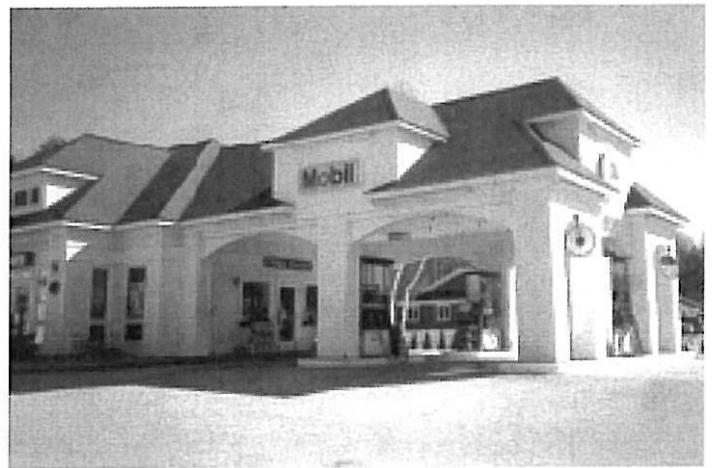
This service station canopy is designed to be an extension of the building. The columns, roofline, details, and signage contribute to a sense of continuity in the architecture.
