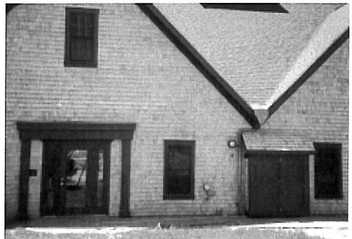
The building's meters and service connections are located out of sight in this service cabinet.
