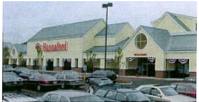
Examples of large retail buildings that have been effectively designed to avoid the appearance of a 'big box'.
