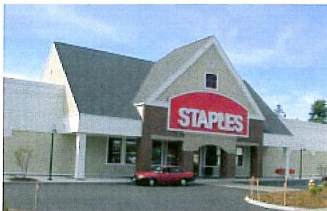
The scale of this 'big box' has been effectively reduced by architectural elements and detailing. The overhang provides protection for pedestrians and emphasizes the entrance.
