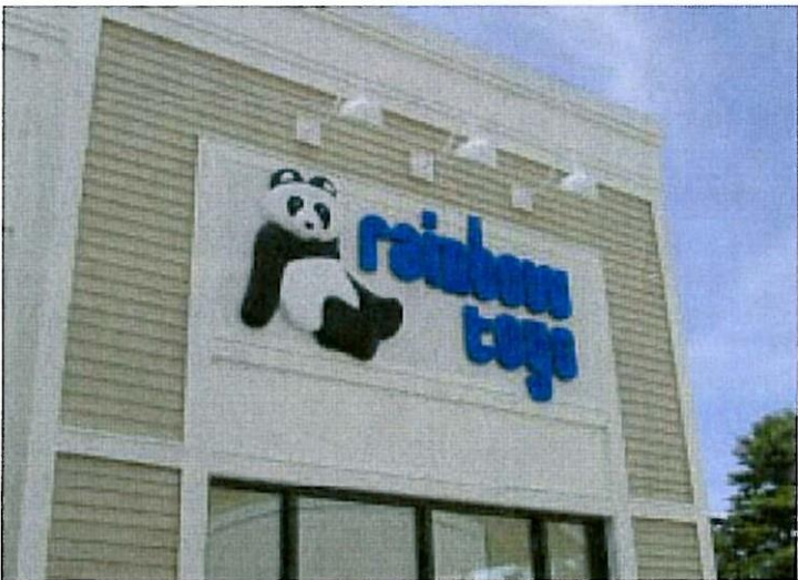
These signs achieve compatibility through the repetition of form, detailing, and materials.
