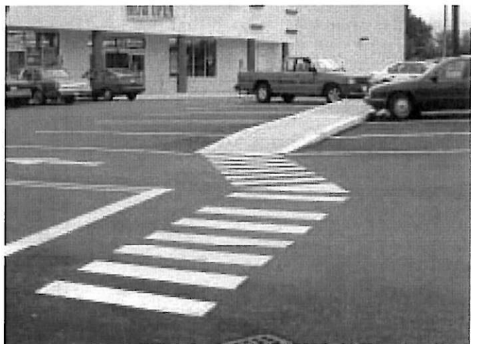
This raised walkway provides a high level of contrast with the surrounding parking lot. However, the width is compromised by the overhang of cars, making pedestrian movement difficult.
