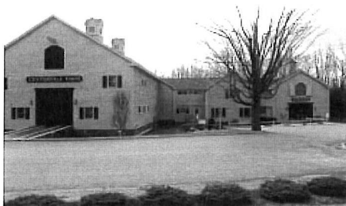
Drawing from traditional forms, the scale of this commercial building is reduced by variations in roofline, massing, and high-quality architectural details.
