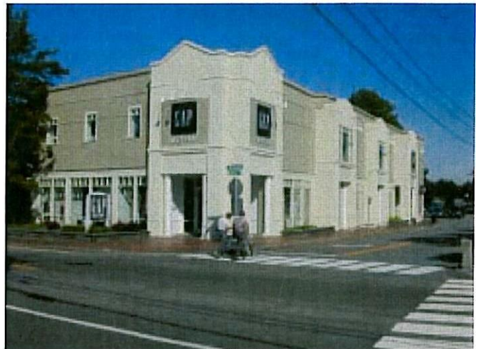
A retail building that is well-sited in its corner location. Attention to design detail gives the building human scale and visual interest.
