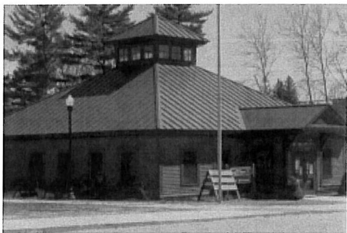
Standing seam metal roofing is a traditional material common in older commercial buildings in New England.
