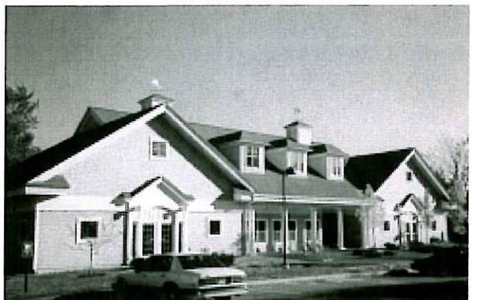
Examples of high-quality Maine architecture -a medical office, a retail store, and a library -that have been designed at human scale and fit their unique sites.
