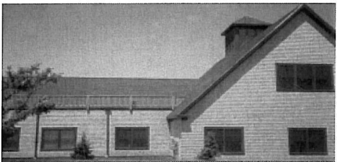
A cupola projecting from this steeply pitched roof is an example of traditional forms used in a contemporary structure. Roof-mounted mechanical equipment has been effectively screened by balustrades.
