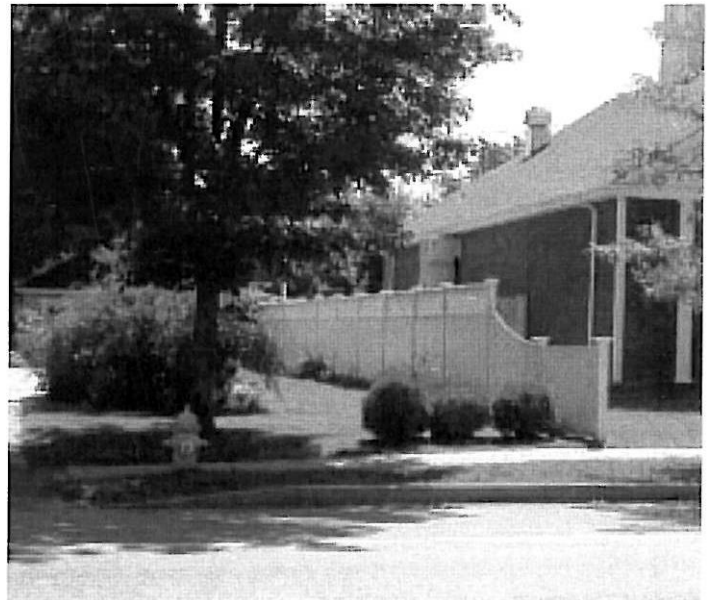
A variable height fence used to provide visual separation between a convenience store and its residential neighbor. The fence is attractive on both sides.
