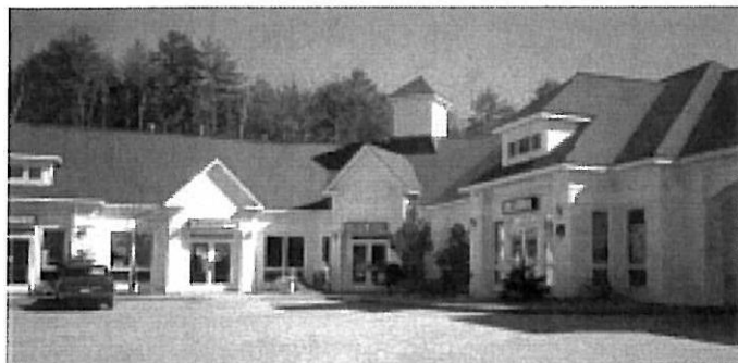
The scale of this linear shopping plaza has been effectively reduced through variations in roof planes, dormers and a cupola.
