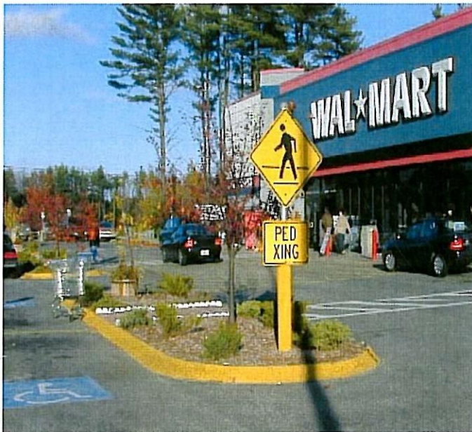
This internal walkway crosses over a curb, making access difficult for people with disabilities.
