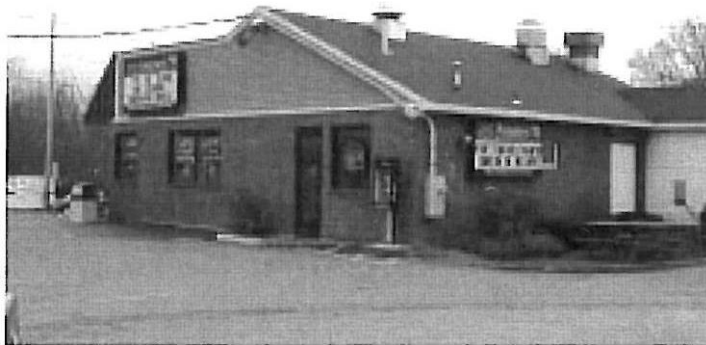
This building & ventilation equipment and service connections are highly visible, adding unnecessary clutter
