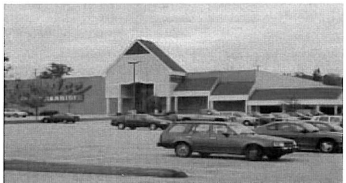
A large retail establishment that still projects the image of a big box, despite the canopy and entrance treatment.
