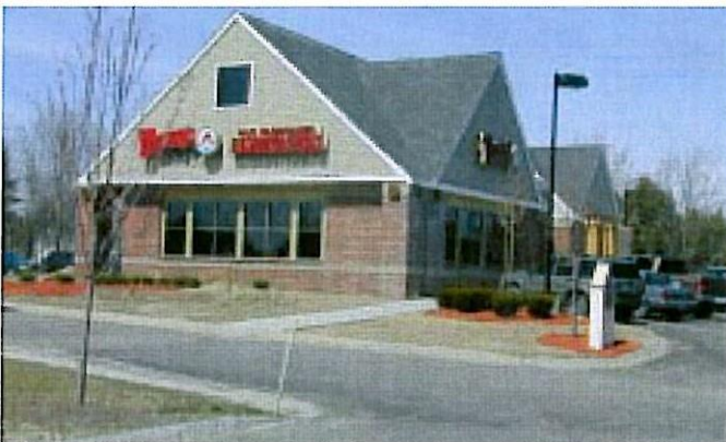
This fast-food restaurant is an 011parcel of a larger commercial retail development. Circulation, including drive-through, parking, and pedestrian access, has been carefully integrated into the surrounding site.
