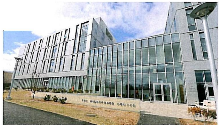
Each of these buildings exhibit predominately flat roofs, but the roof lines vary with the introduction of different roofline elevations and screened roof top equipment and mechanicals.
