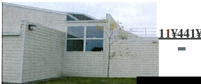
Cement plank clapboard is a new material that resembles traditional wooden siding with less maintenance.
