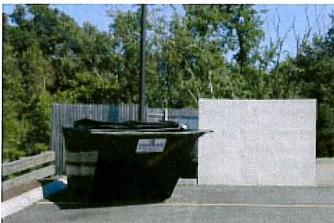
This trash enclosure was not properly sized to handle the dumpster needed for the facility.
