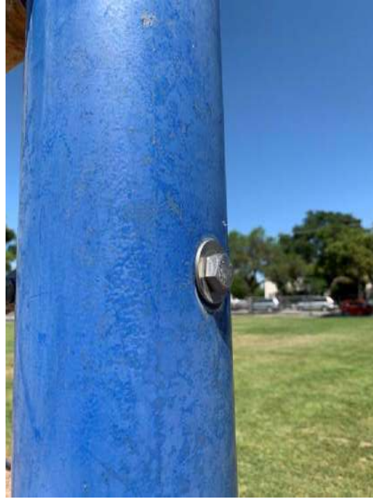
Bolt protrusion.
