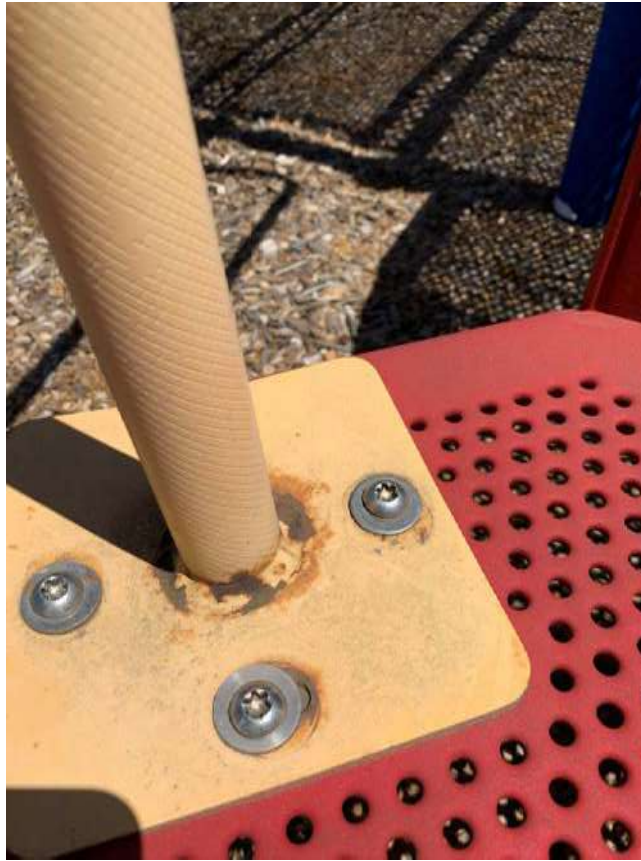
Rusty edges and corrosion of metal pieces, fasteners, and clamps.
