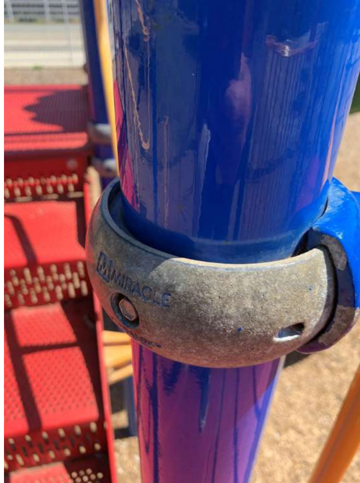
Corrosion on fasteners and clamps.
