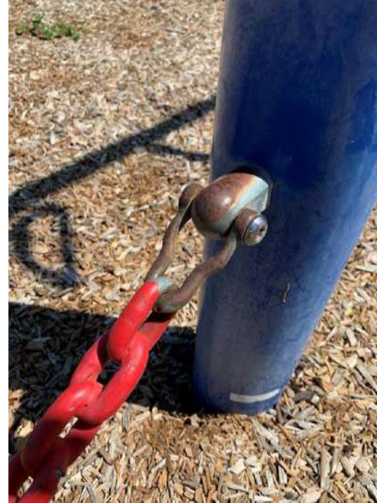
Corrosion evident on hardware and chains
