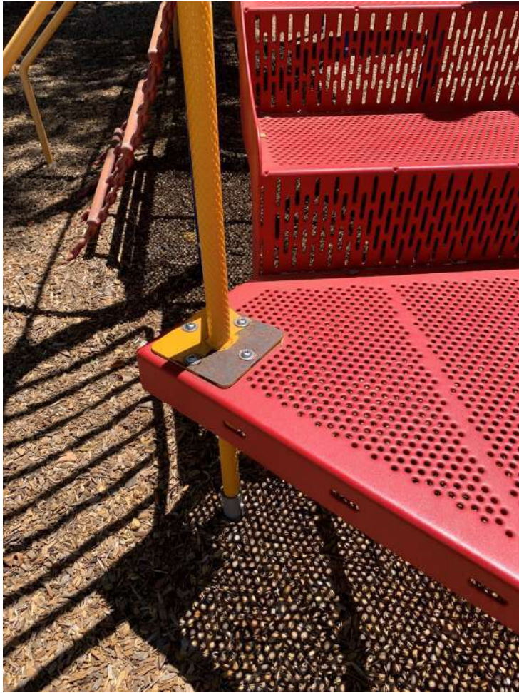
Transfer station missing step.
