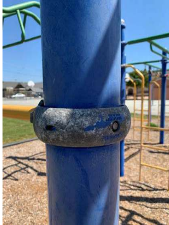
Corrosion on metal support clamps.
