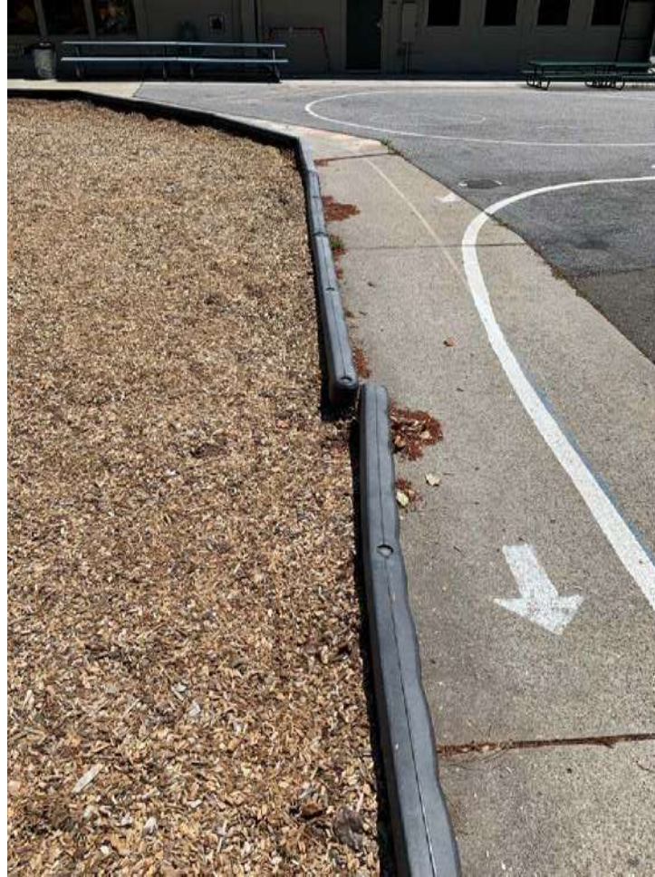
Wood fiber containment borders failing.
