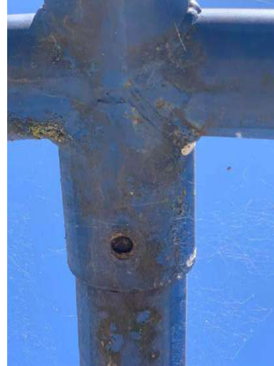
Corrosion evident on metal components. Missing hardware.
