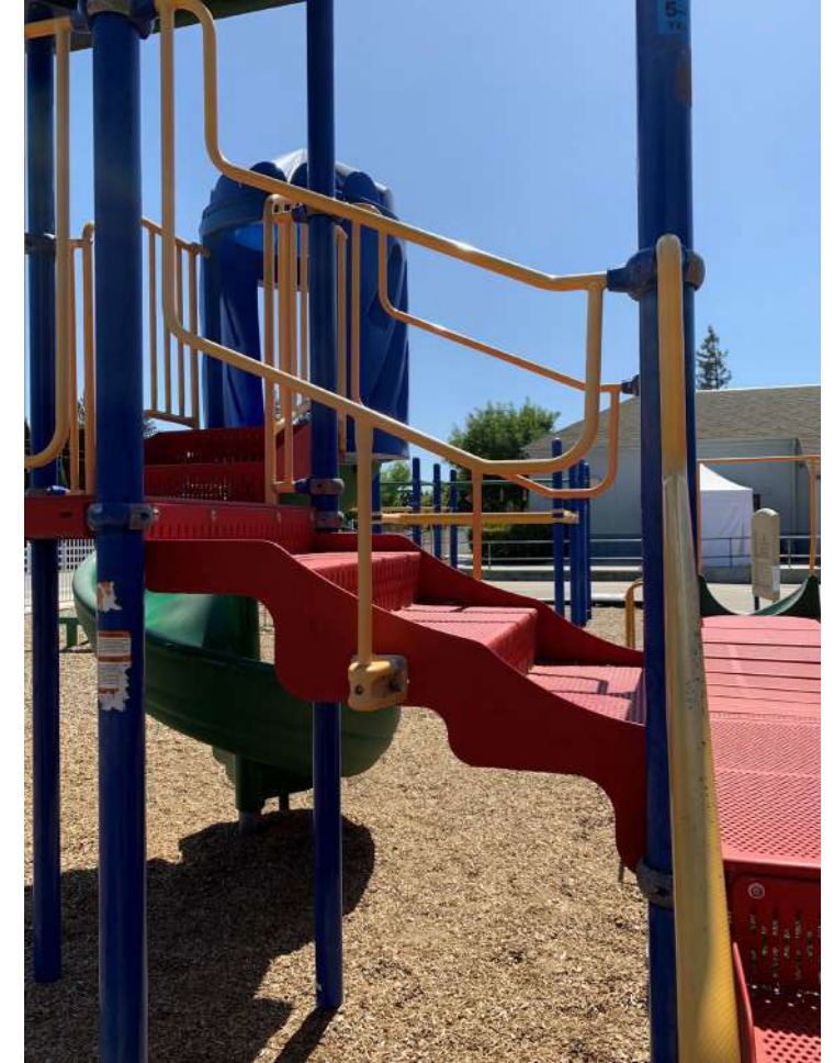
Railings not compliant if used by children under 5 years old.
