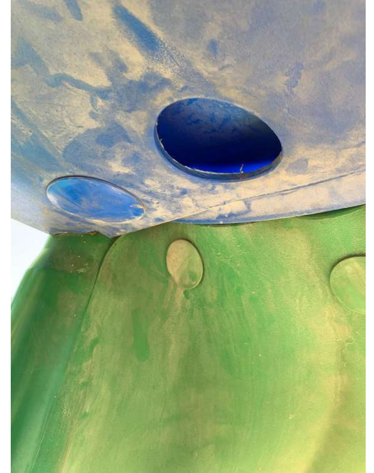
Holes in plastic slide allow place for insects to nest.
