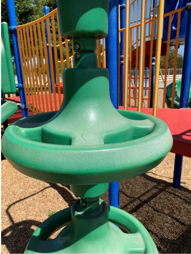
Loose on post and footing.
