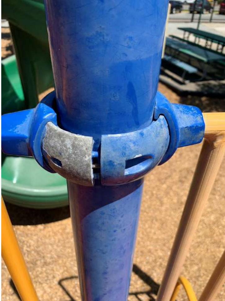
Support Clamps broken and pulling apart.
