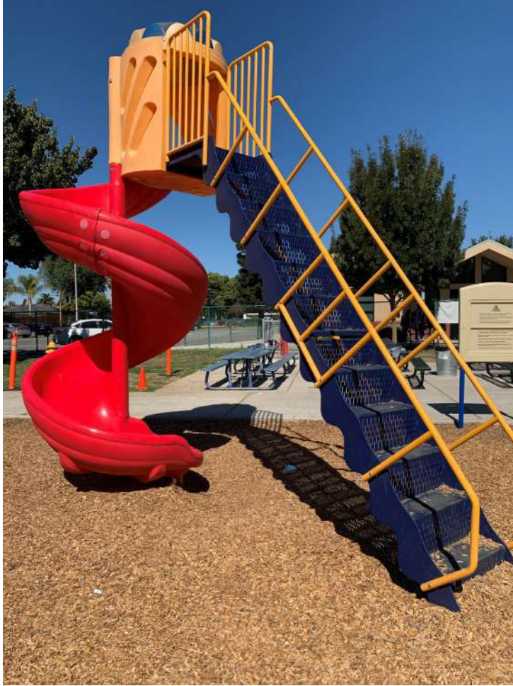
Non-Compliant Railing on Stairs.
