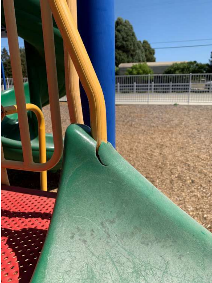
Broken Slide: Entanglement and laceration hazard.
