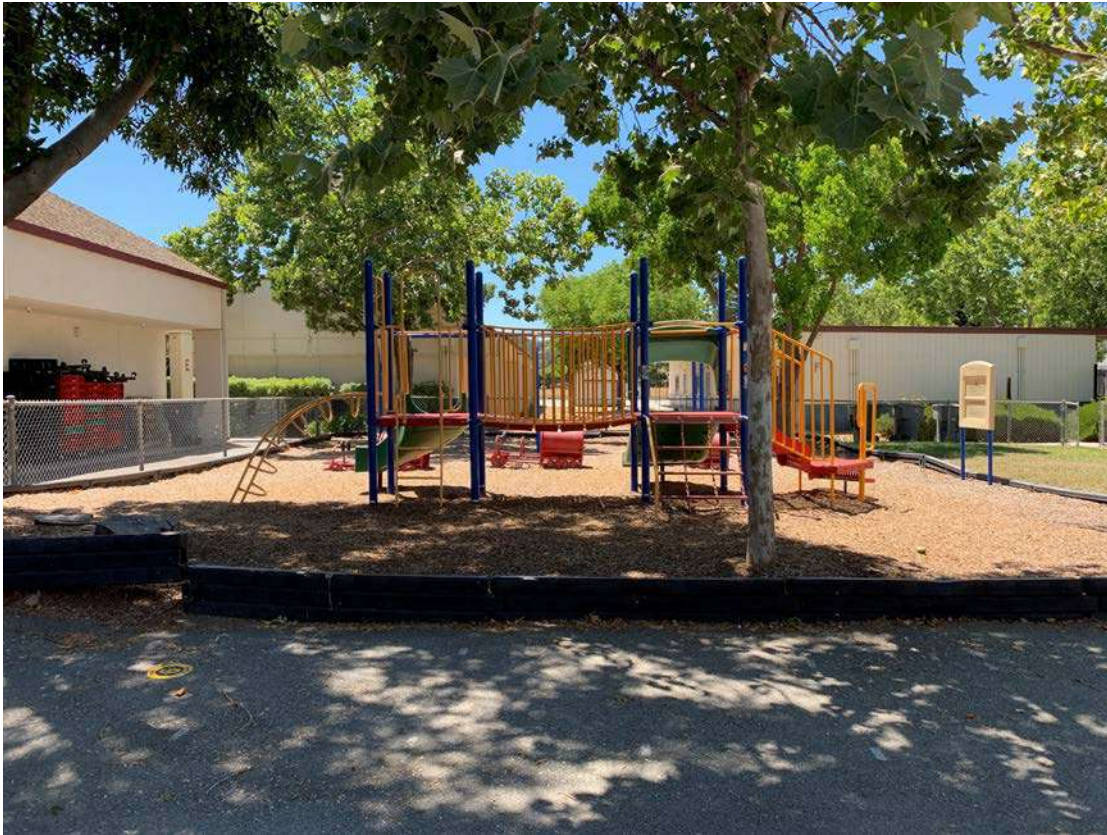
Borders failing due to tree roots and no ADA access to box.
