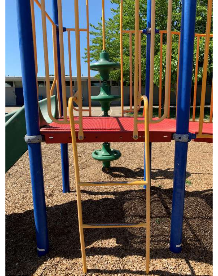
Bent/warped ladder.
