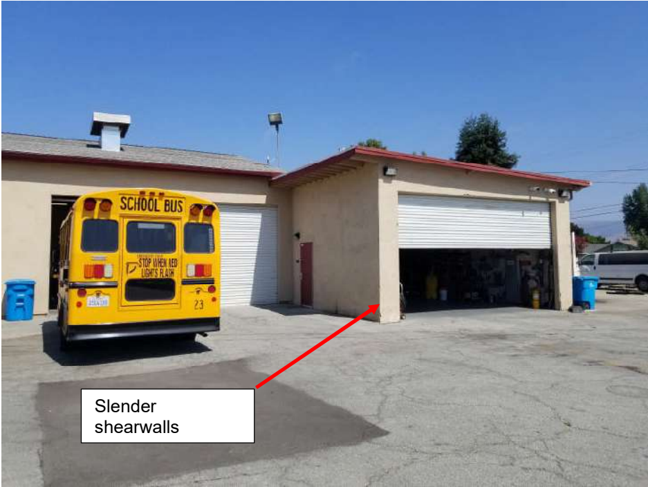
Figure 8 – Building 100 eastern shearwalls
