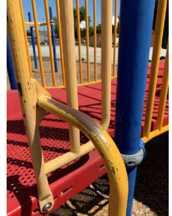
Corrosion and wear on handrails and climbing elements.
