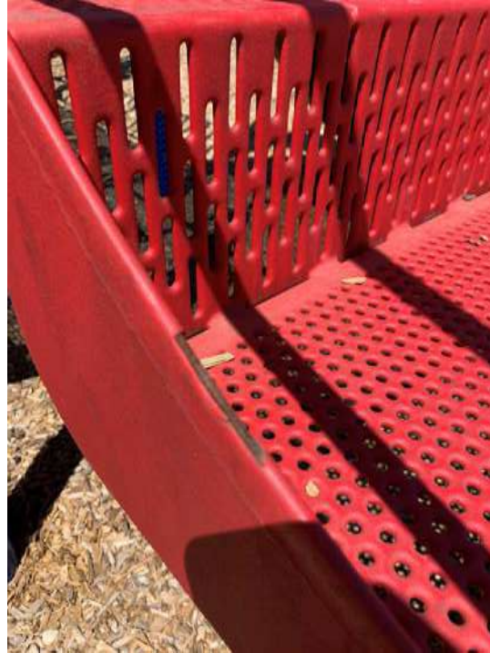
Exposed rusted edges on stairs.
