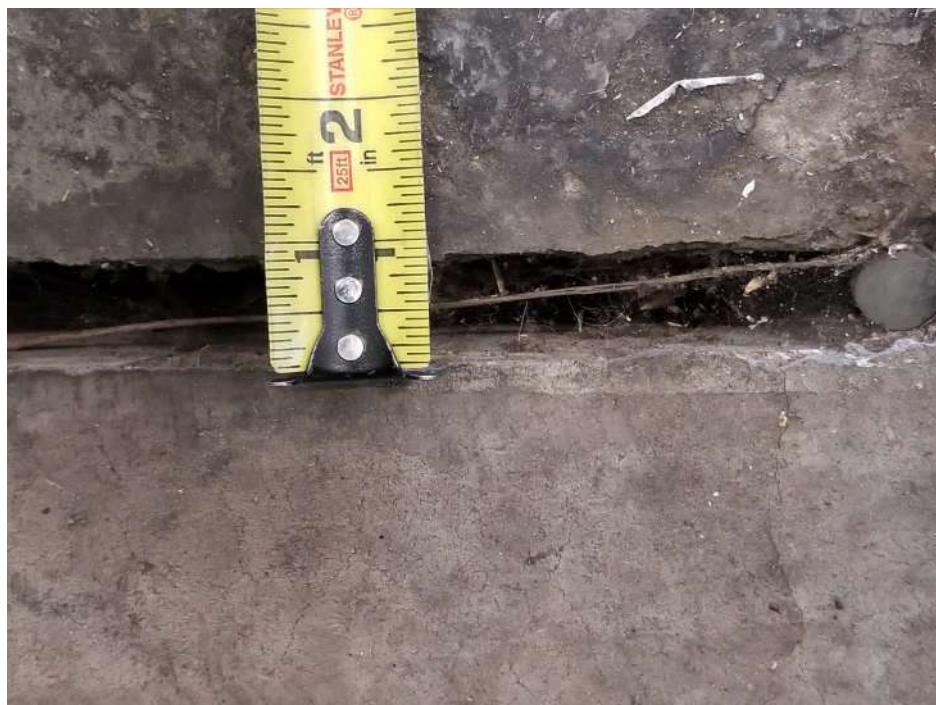
Figure 4 – Crack in rear of Building 100
