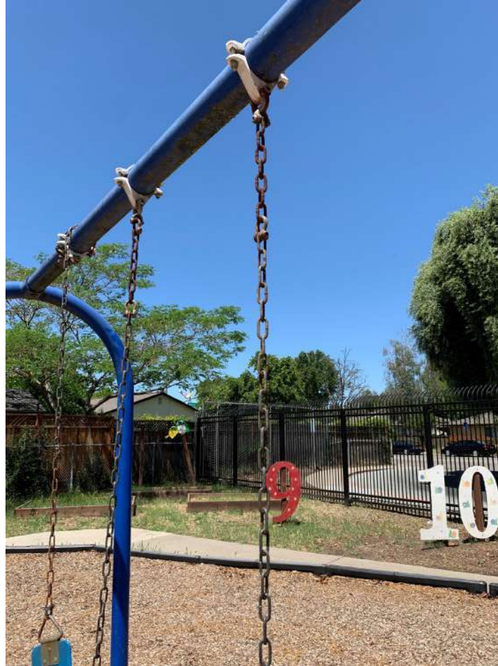
Swing chains joined by quick links and clevis mid-chain.
