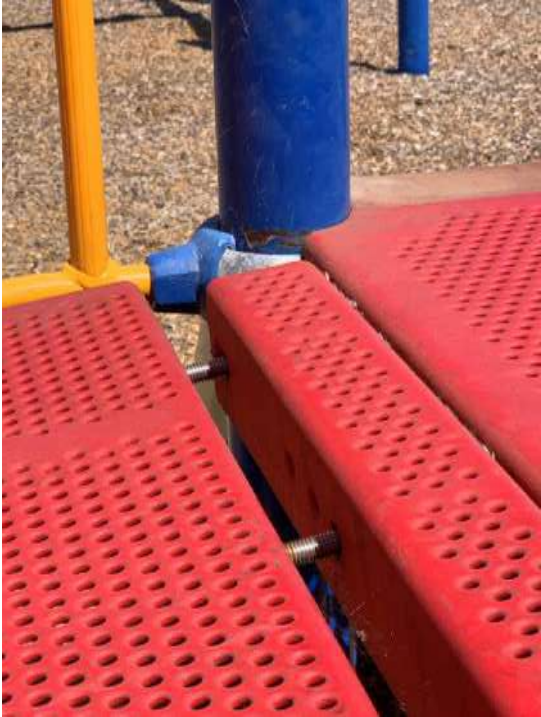
Severe corrosion of post and gap too wide at clatter bridge.
