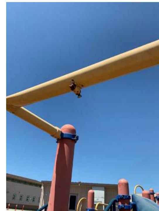
Missing equipment and broken hardware at “pod” climber poses entanglement and is non-compliant for distance from pod to deck.
