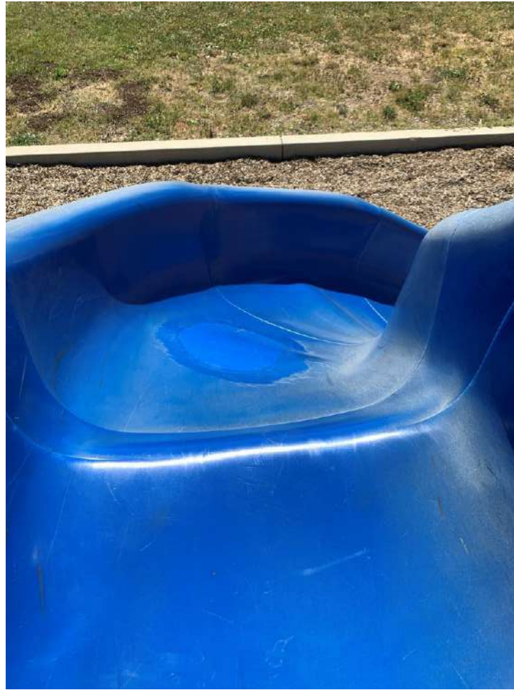
Sectional Slide warped and Bumpy.
