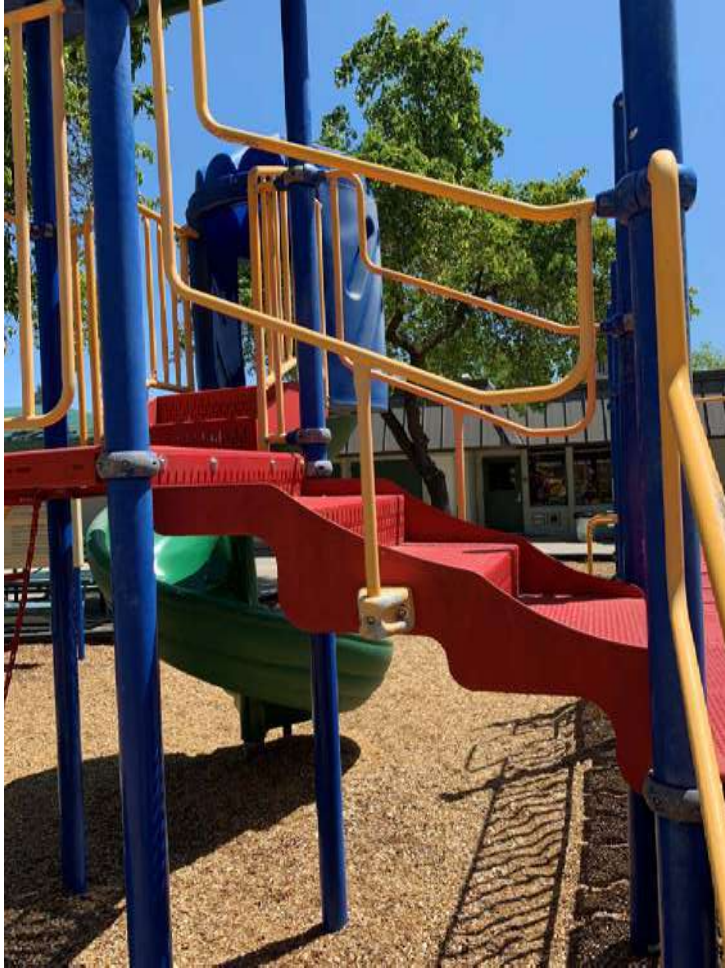
Non-Compliant Railing if used by children under 5 years old.
