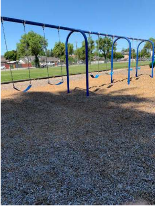
Swing area lacking fall surfacing depth.
