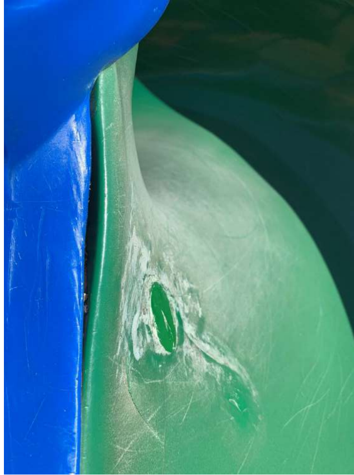
Entanglement Hazard at spiral slide entry.
