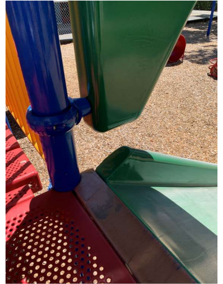
Potential partially bound neck entrapment.
