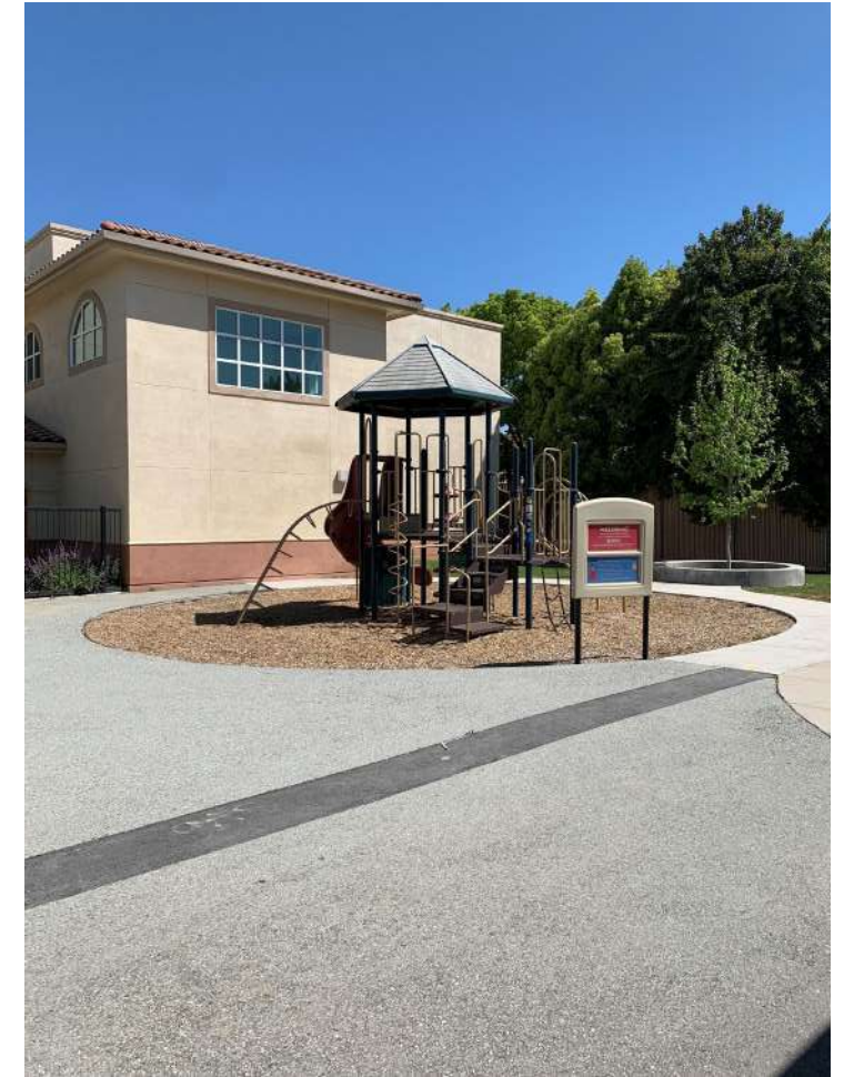
No ADA ramp access into play box.
