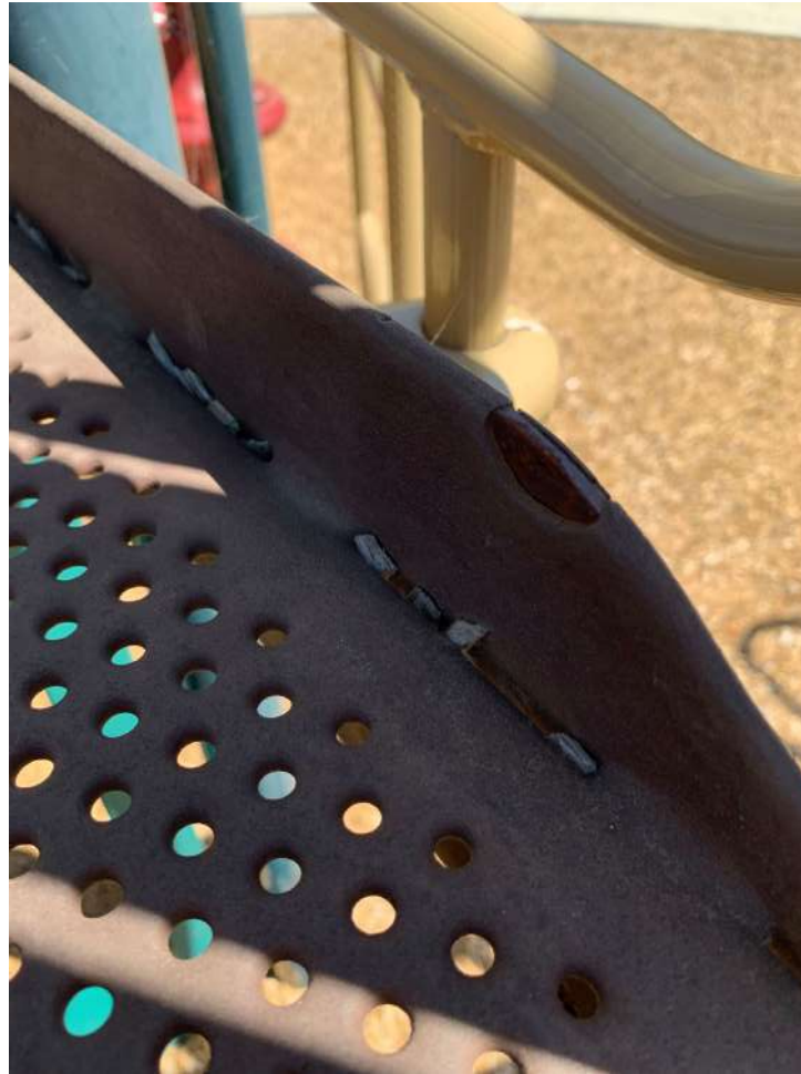
Exposed rusty edges on stairs and decks.
