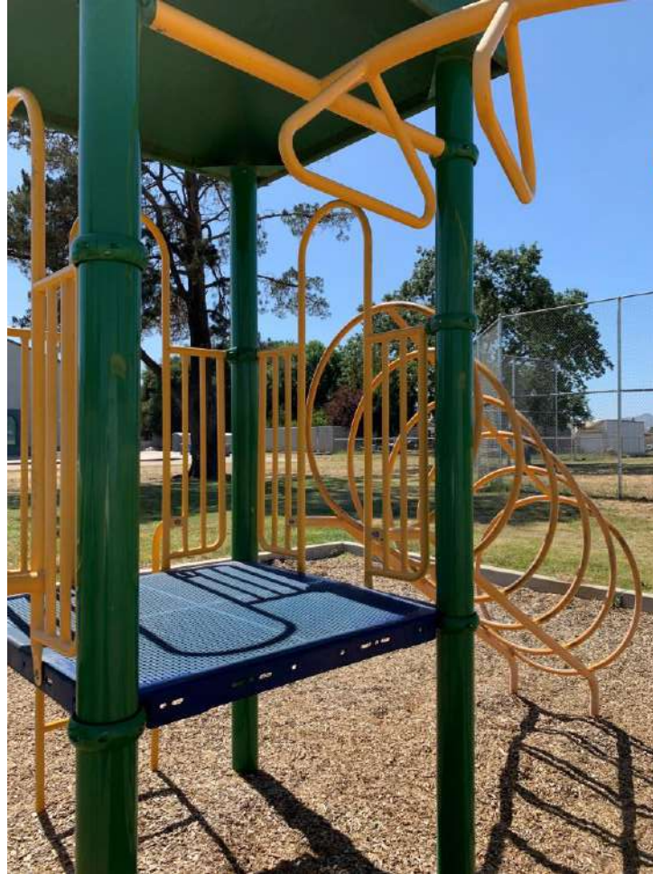
Entry point from Deck to overhead climber not compliant.
