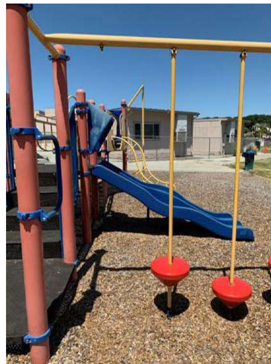
Missing equipment and broken hardware at “pod” climber poses entanglement and is non-compliant for distance from pod to deck.
