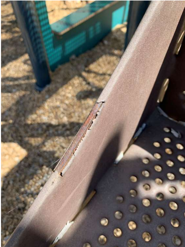
Exposed rusty edges on stairs and decks.
