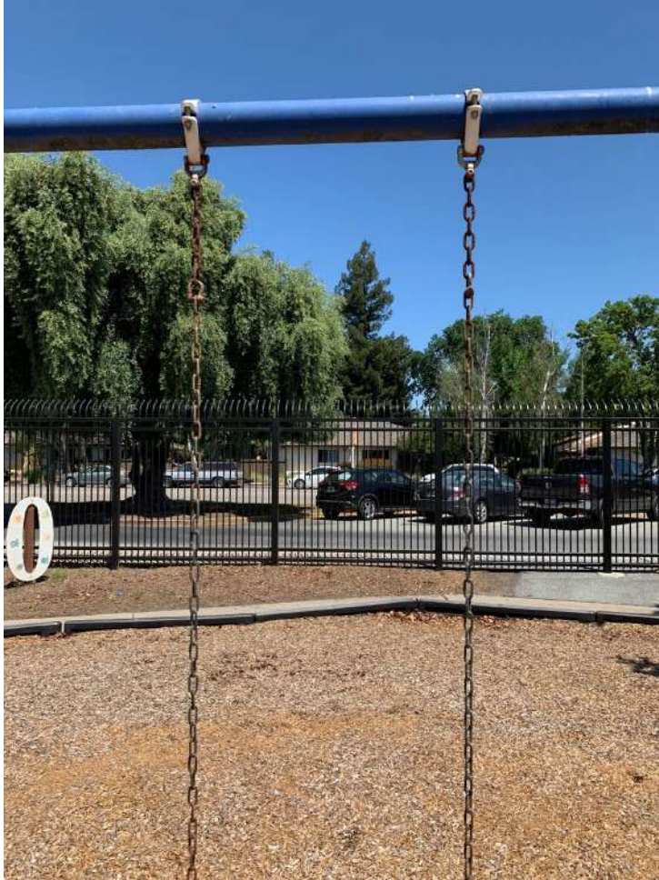
Swing connection points aged and showing signs of corrosion and deterioration .
