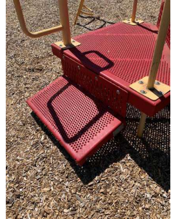
Broken ADA transfer Step.
