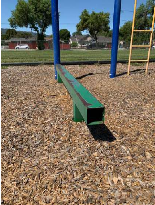
Rusted balance beam with open, sharp edges. Providing insects place to nest.
