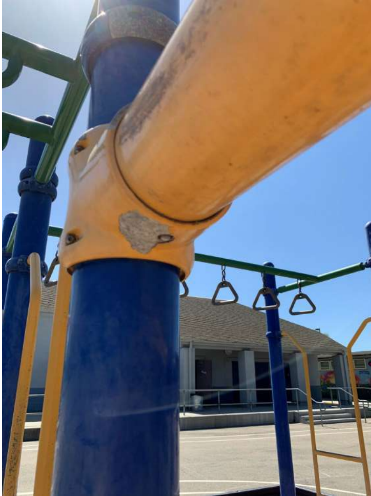
Corrosion and mold evident.
