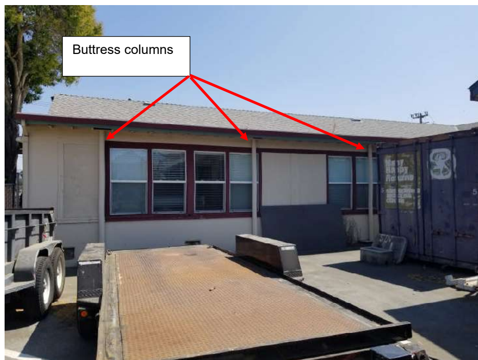
Figure 9 – Building 400 buttress columns
