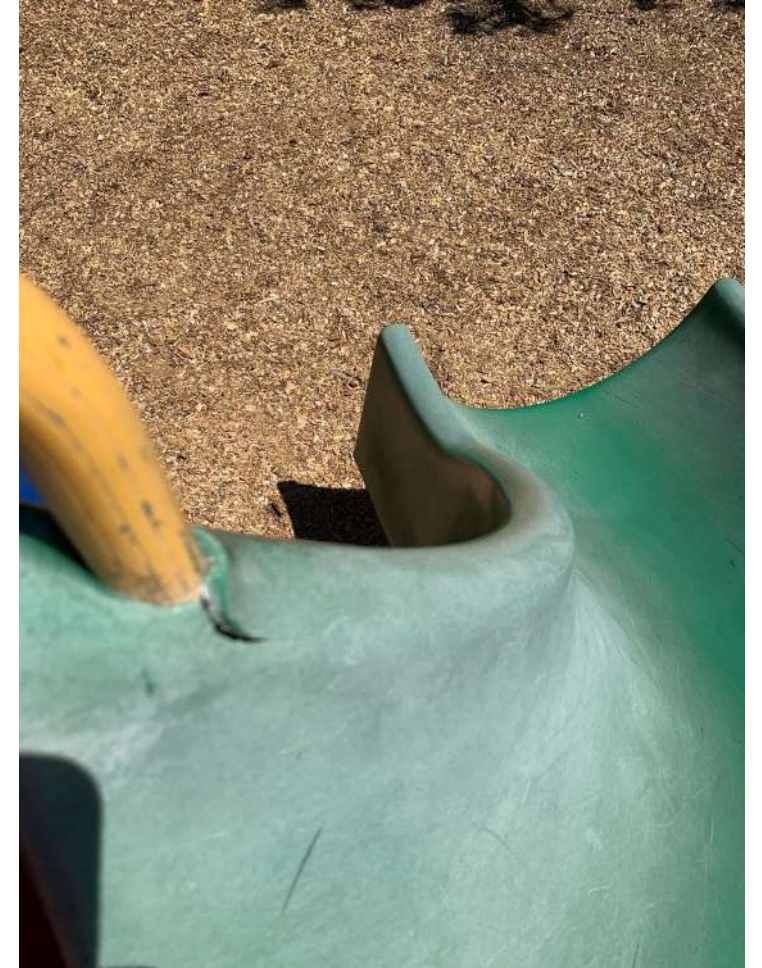
Slide Broken-Entanglement and laceration hazard.
