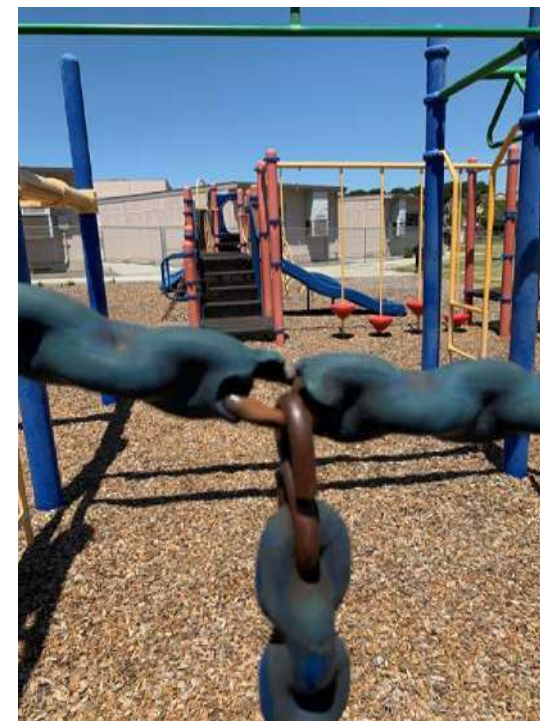
Open “S” hooks used on other connecting climbing elements. Rusted and potential entanglement.
