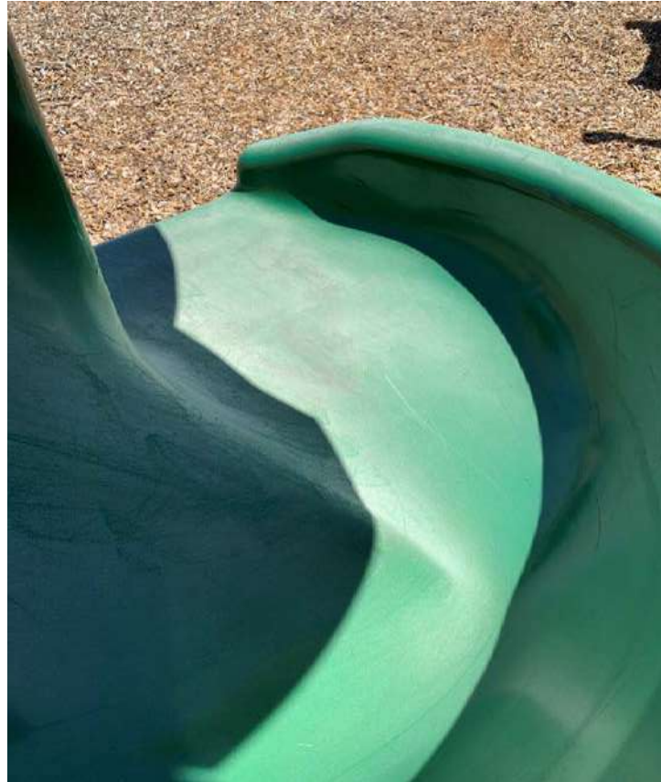
Deterioration of plastic slides make slides rough and scratchy and lumpy.
