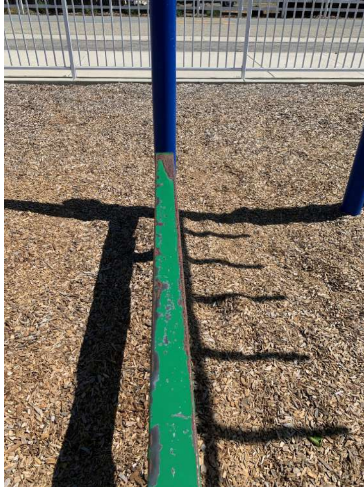
Rusted balance beam.
