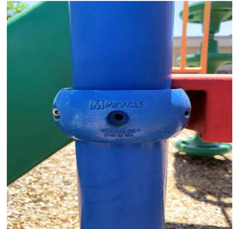
Missing bolts from support clamp
