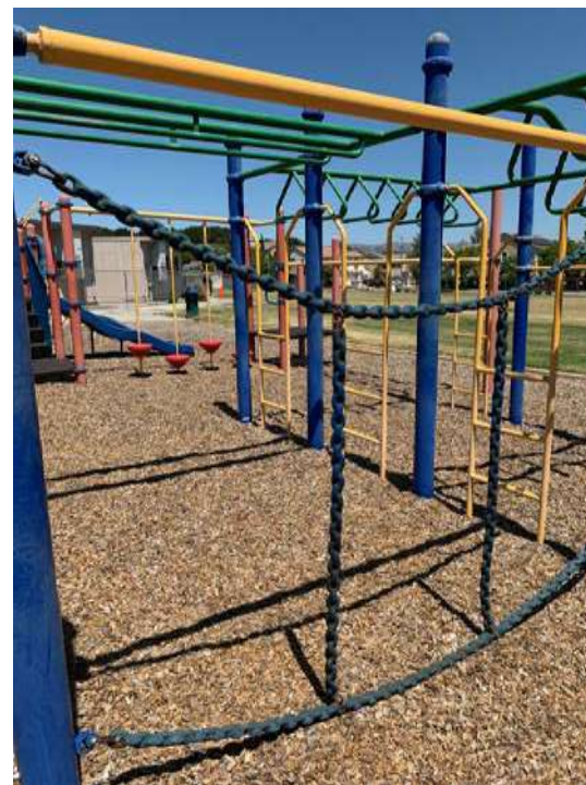
Open “S” hooks used on other connecting climbing elements. Rusted and potential entanglement.
