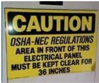
Electrical hazards can be found throughout performing arts operations and include, but are not limited to, exposed wiring, improperly spliced wires, improperly installed temporary power distribution, improperly grounded wiring, use of damaged electrical cords, and the use of inappropriate size and type of extension cord.
