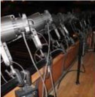
Performing arts lighting rigs are very heavy and can cause severe injuries if they fall. Employees and students must be trained on how to hang and properly secure lights. All lights must be tethered to the lighting rig with a safety cable and double-checked for safety.
