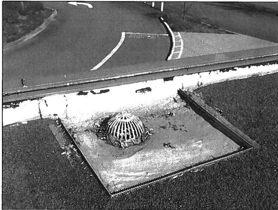
HE. 1.05 – View of typical roof drain and overflow scupper at the northwest section of the roof.
