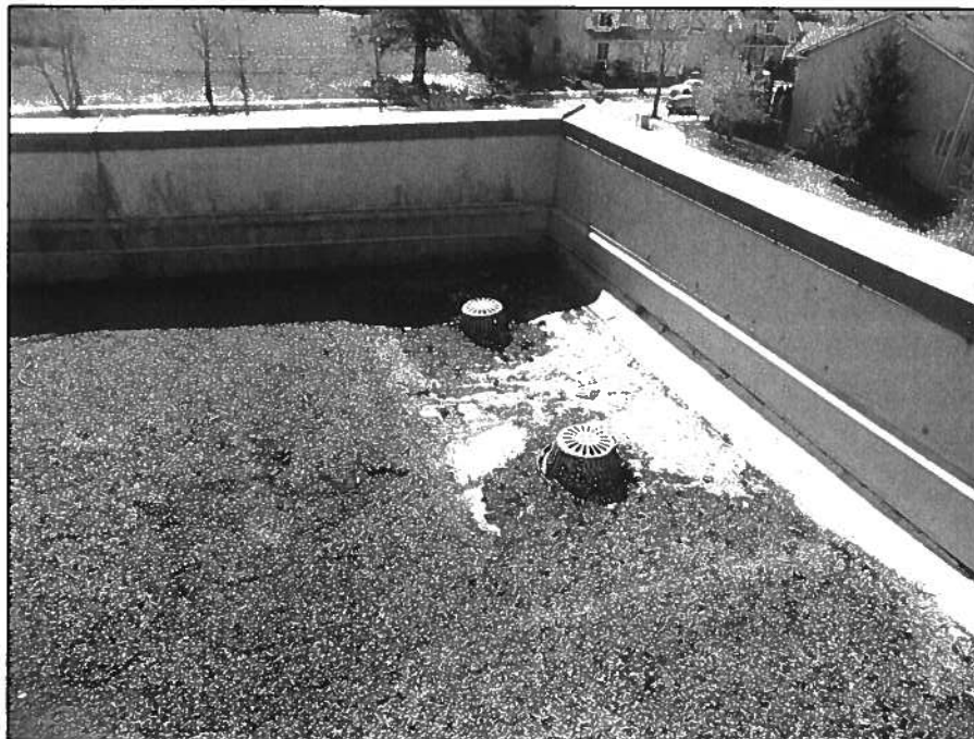
JWE. 1.04– View of typical roof drain and overflow drain at the west section of the roof.
