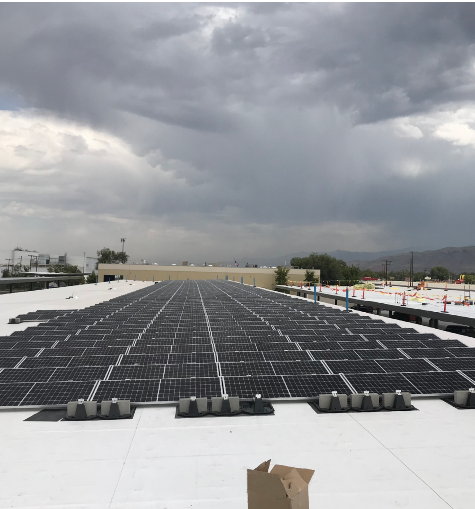
200 kW photovoltaic solar array on school bus protective canopy.
