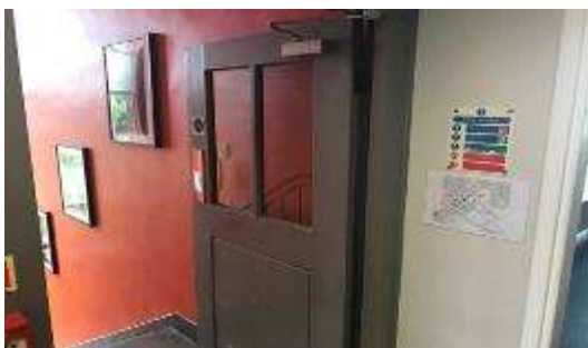
Fire doors requiring adjusting throughout
