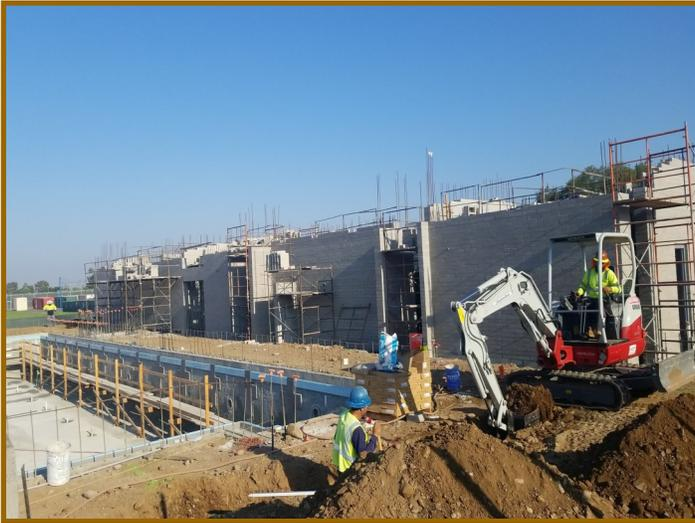
Construction on El Modena High School's Aquatics Center continues at a fast past. Tile is currently being added to the new 30-meter pool. Block construction is nearly complete on the 3,000 square foot locker room/pool equipment building with roof structure installation scheduled to begin in September 2021. The Aquatics Center is on track to open in Spring 2022. The project is being paid for by the District's special capital outlay reserve fund which is funded by the sale of surplus property.
