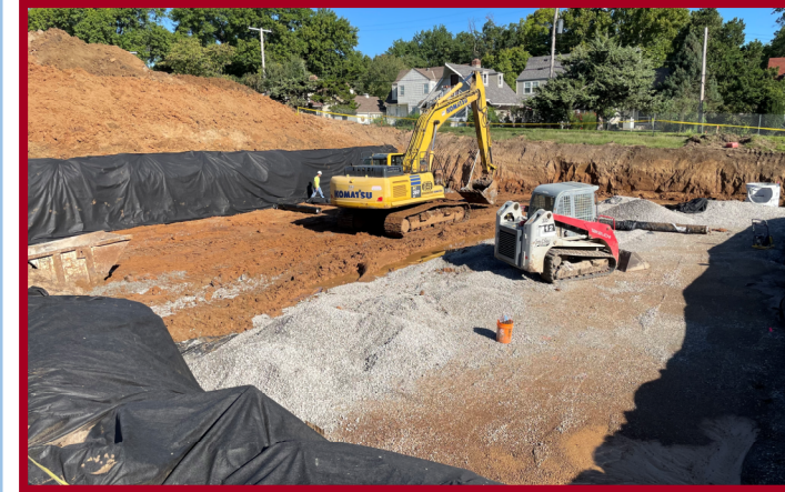
Underground Detention Basin Excavation
