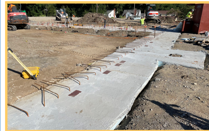
Gym Footings & Precast Embed Plates
