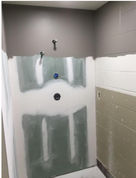
Toilet 121 Shower Rough-in
