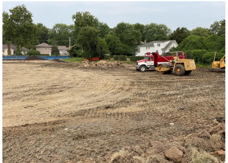
North Side of Jobsite
