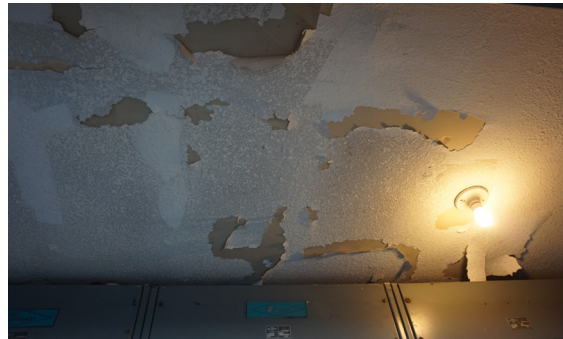
Ceiling condition in maintenance rooms.
