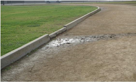
Puddling and drainage issues on track.
