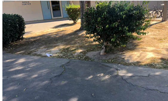
Cracking caused by plants roots.
