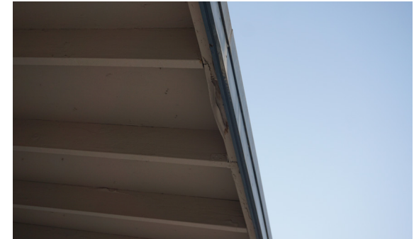
Damaged/rotting fascia boards.
