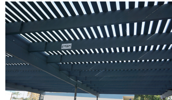
Wooden shade structure needs to be replaced.
