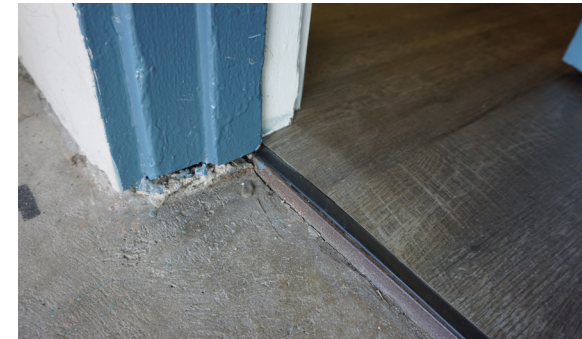
Cracked, uneven thresholds into classrooms.
