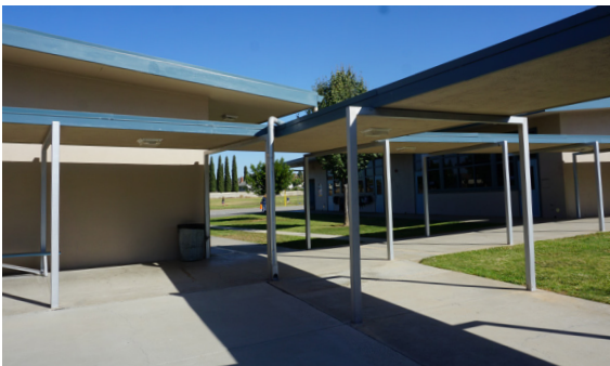
Typical covered walkway.
