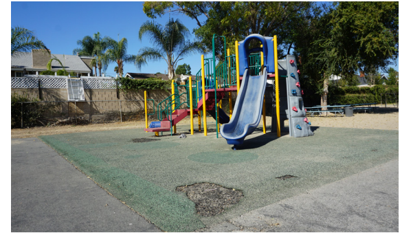
Play structure ground condition needs attention.
