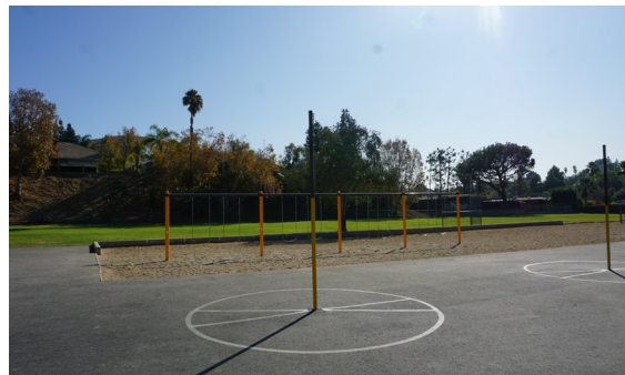
Sand under swings in need of replacement.
