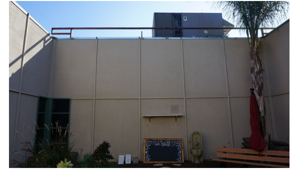
Atrium area adjacent to front office.
