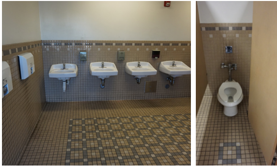
Typical restroom condition.
