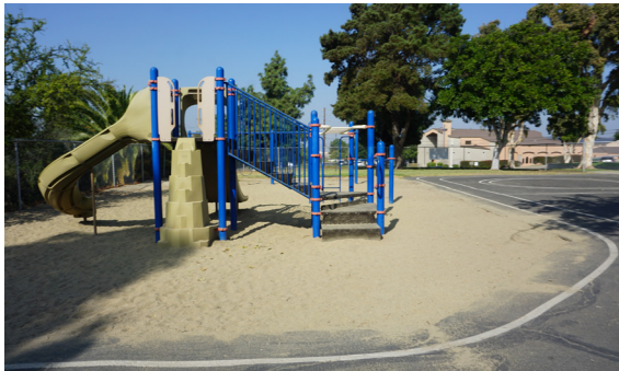
Sand under play structure needs replacing.
