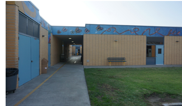
Typical exterior hallway between classrooms.
