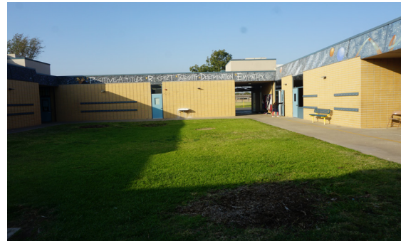
Atrium area outside of main office.
