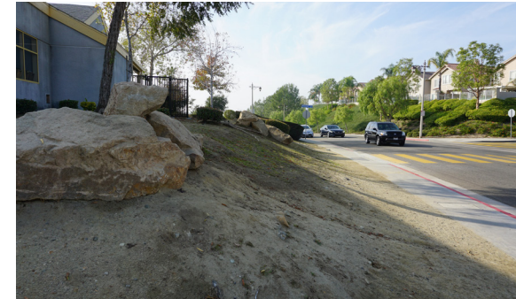
Lack of landscaping causing runoff on sidewalks.
