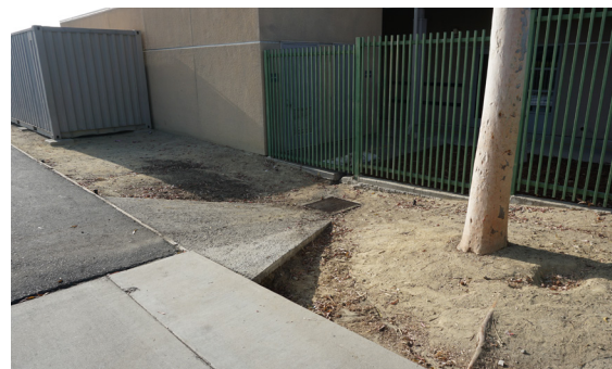
Lack of landscaping around campus.
