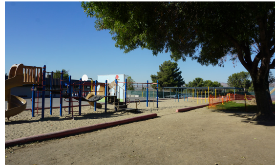
Non-compliant access to play structures.
