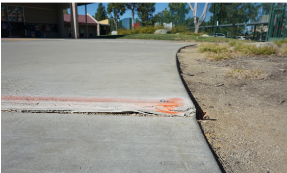
Raised concrete pads.
