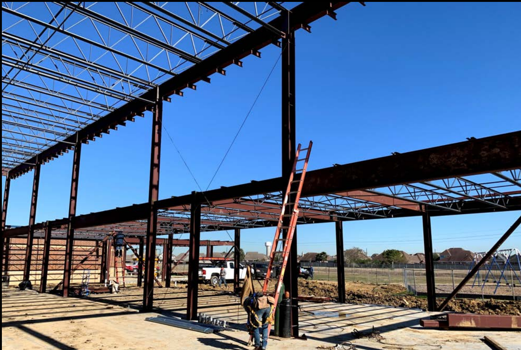
Area C - Library Addition Structural Steel and Roof Joist
