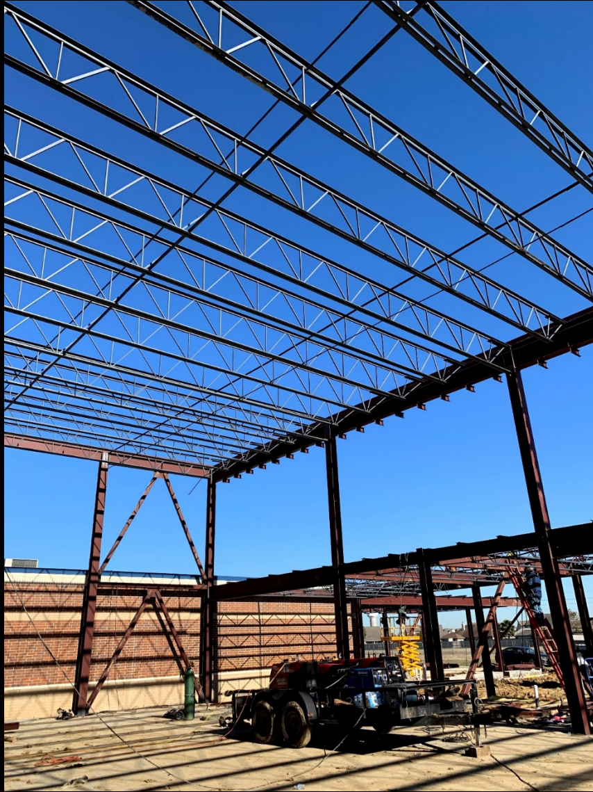
Area C - Library Addition Structural Steel and Roof Joist
