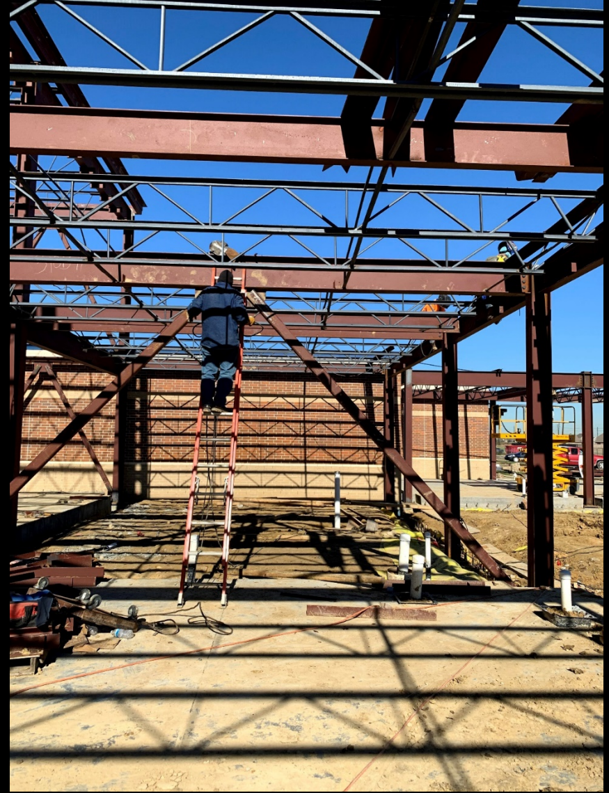
Area C - Library Addition Structural Steel and Roof Joist
