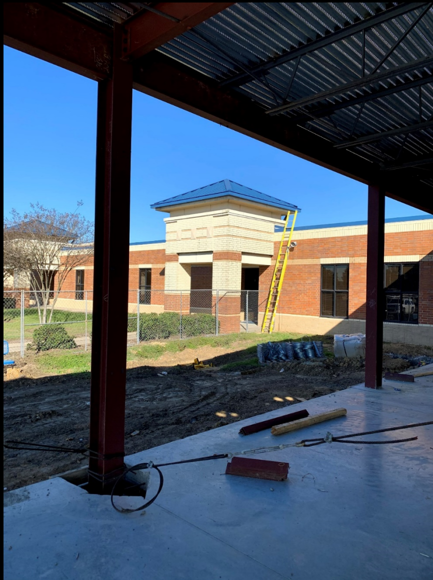
Area B - Classroom Wing Structural Steel & Roof Deck
