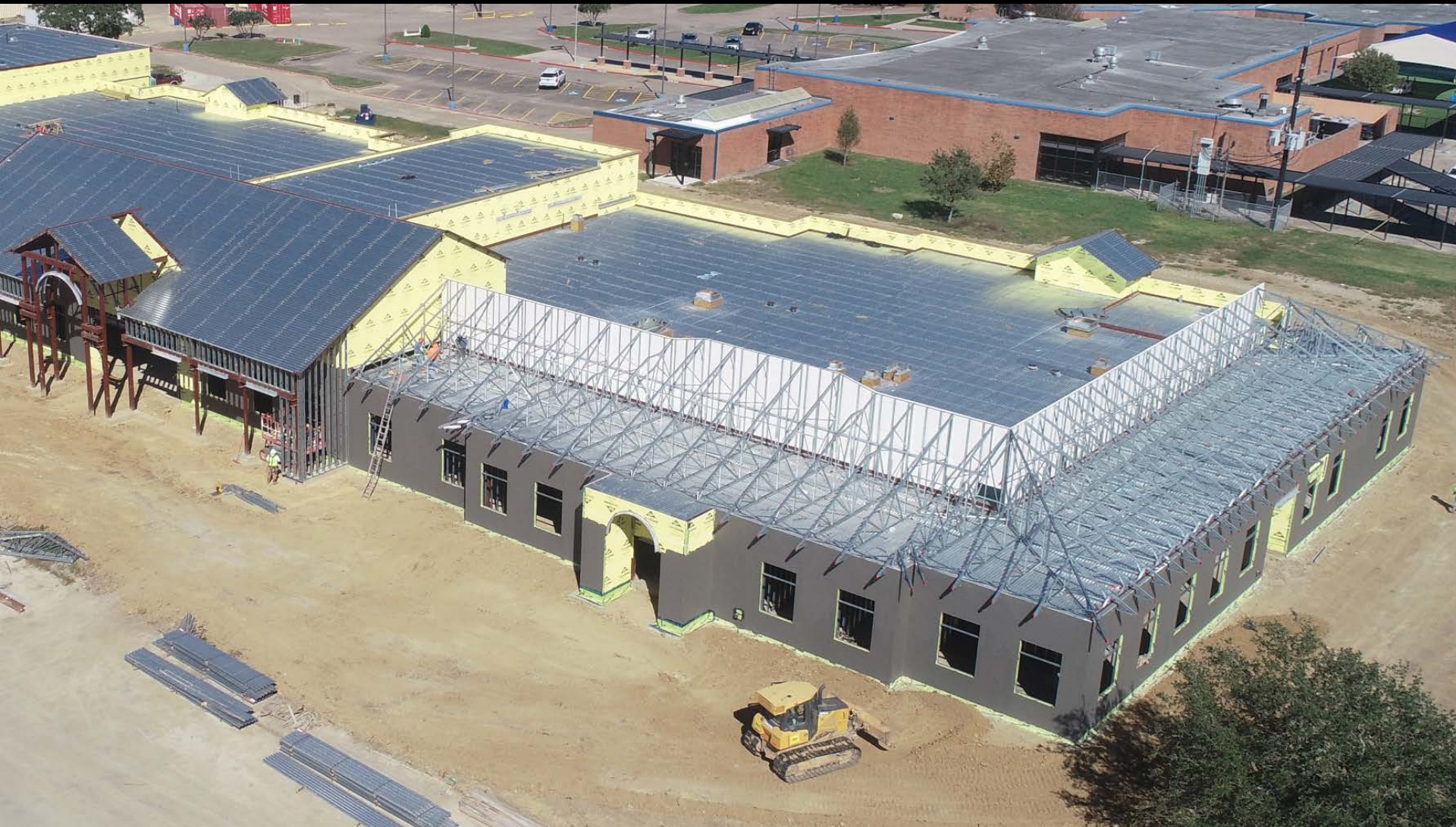
Aerial – Tax Office Entry - Exterior Walls & Roof Decking with Metal Trusses
