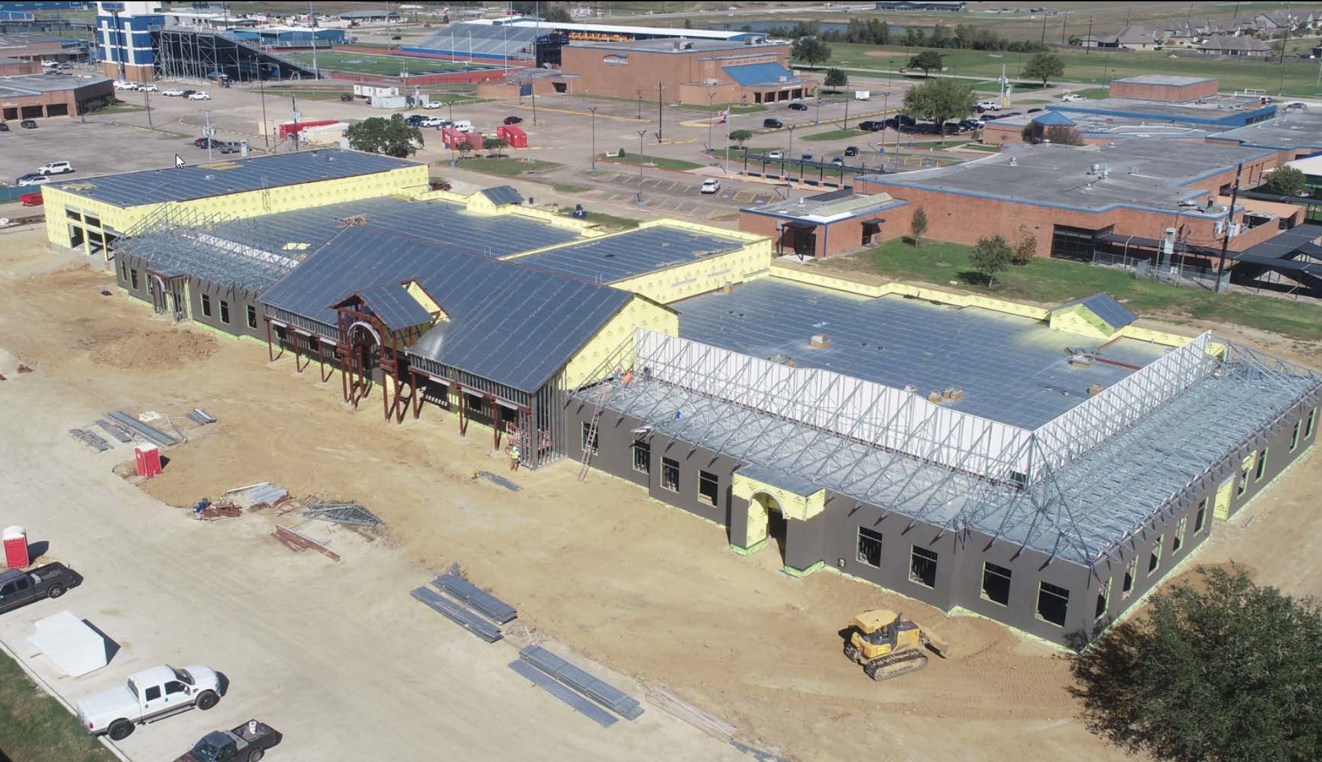
Aerial - Front Elevation - Exterior Walls, Roof Decking with Metal Roof Trusses
