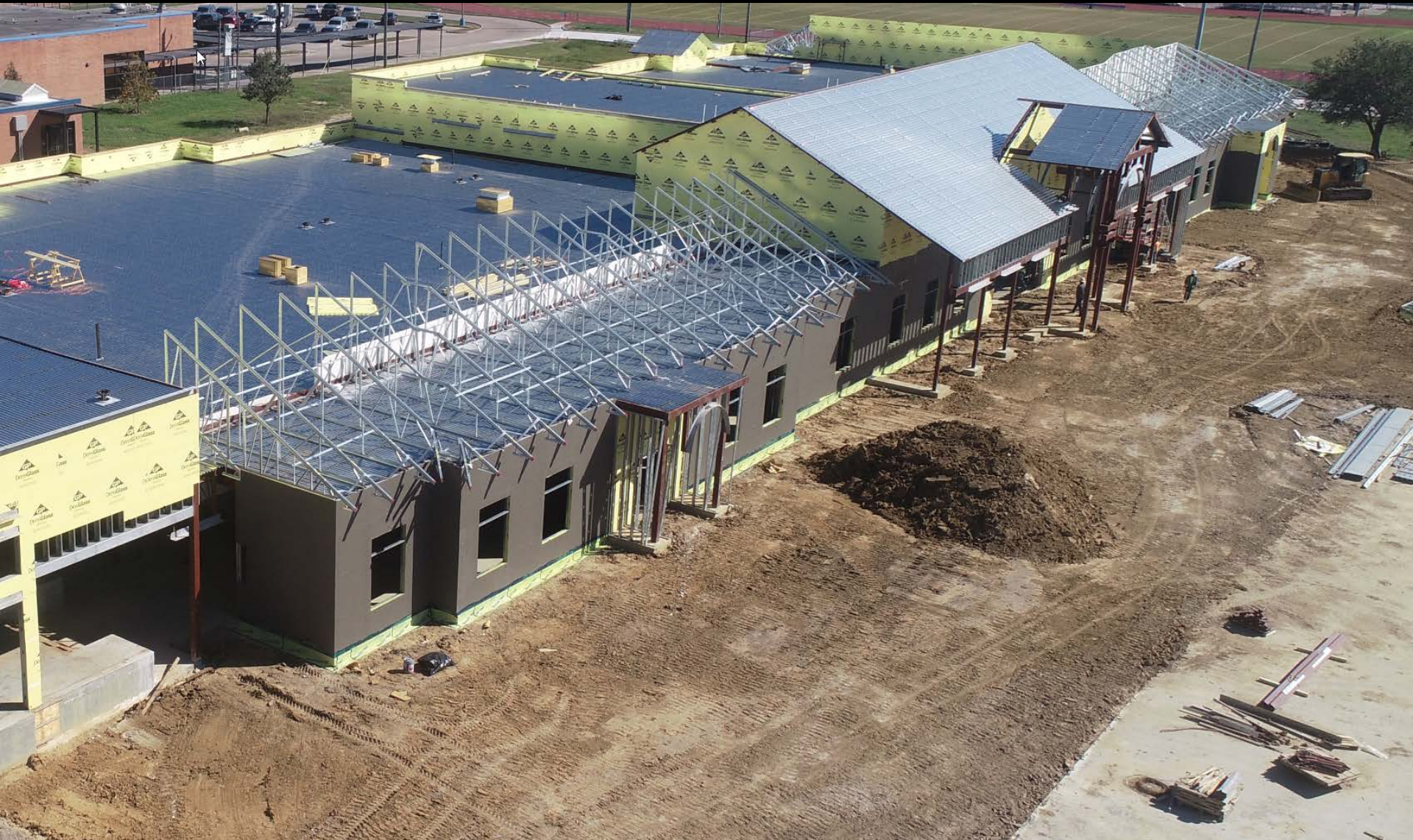
Aerial - Front Elevation - Exterior Walls with Weather Proofing; Roof Decking with Metal Trusses
