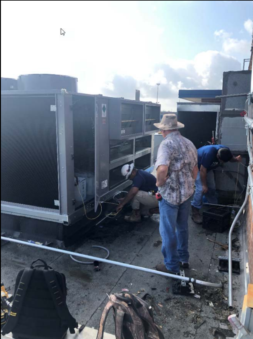
New Roof-Top HVAC Unit Being Installed
