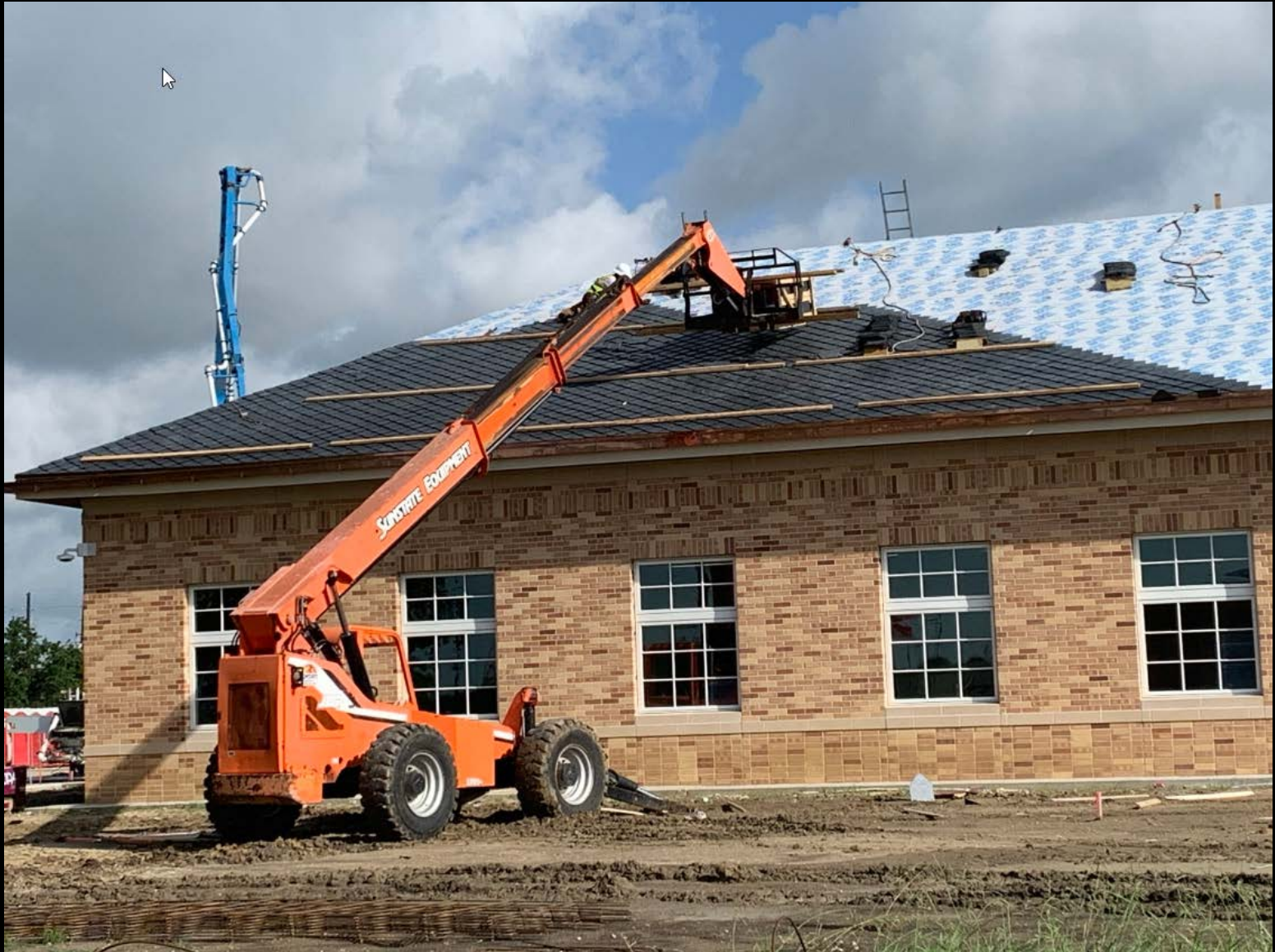
Slate Roof Shingles installation in Progress
