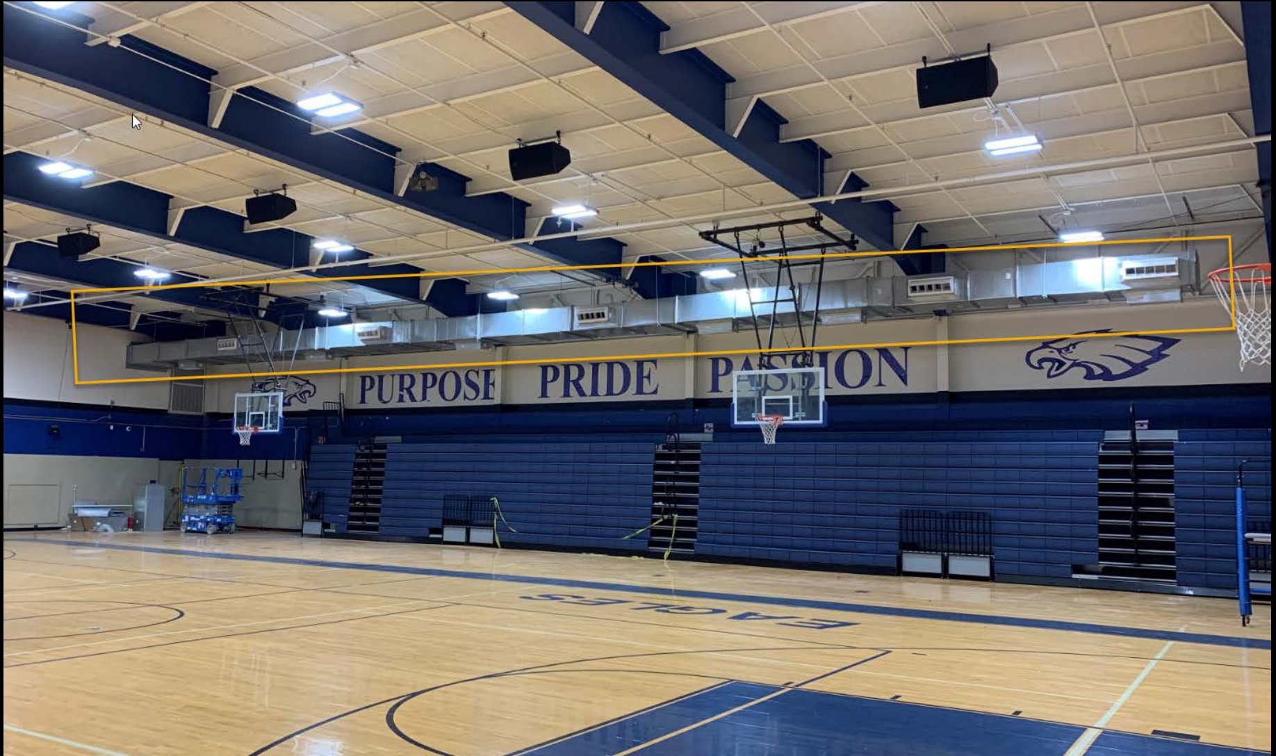
New Ductwork for Southside Roof-Top Unit (before painting)
