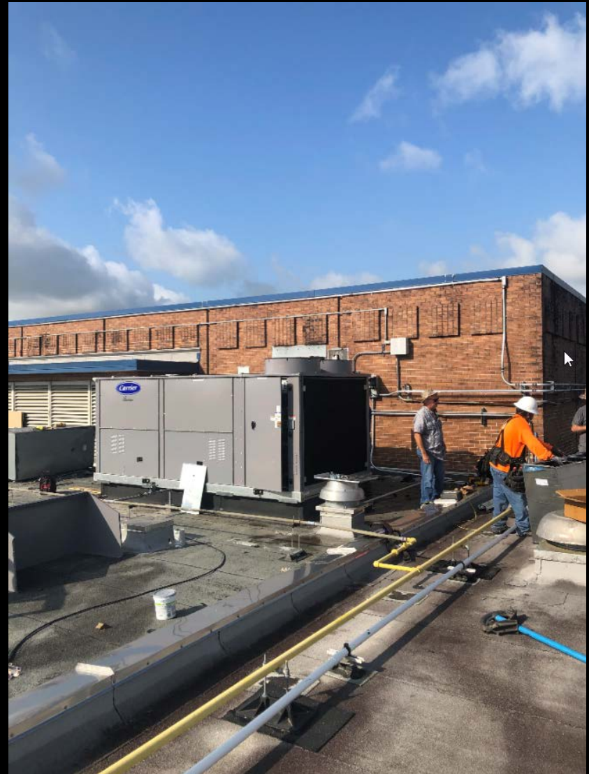
New Roof-Top HVAC Unit Being Installed
