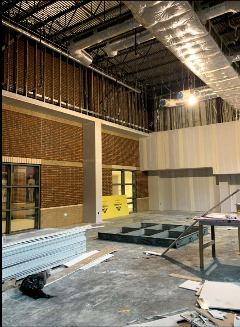
Area C - Library Clearstory – Taping and Floating of Gypboard
