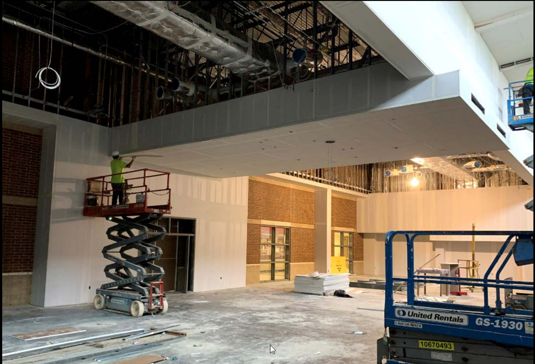
Area C – Library – Taping and Floating of Gypboard
