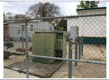
Photo No.12 – Pad-mounted transformer adjacent to Murray Ave.
