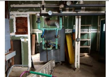
Photo No.7 – Boiler for former swimming pool.
