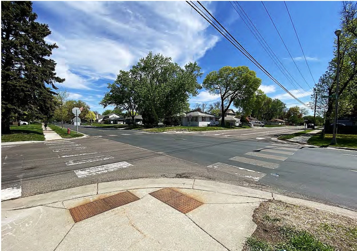
70 th Street and 12 th Avenue intersections looking northeast. Source: SRF Consulting Group, 2020
